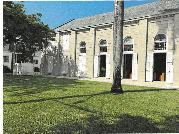
EXISTING PARTIAL WINDSOR SIDE
