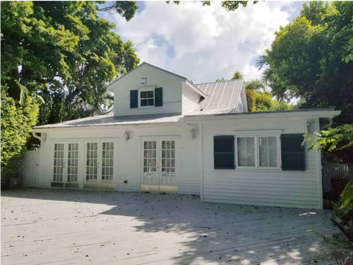
REAR SIDE VIEW OF PRIMARY STRUCTURE
