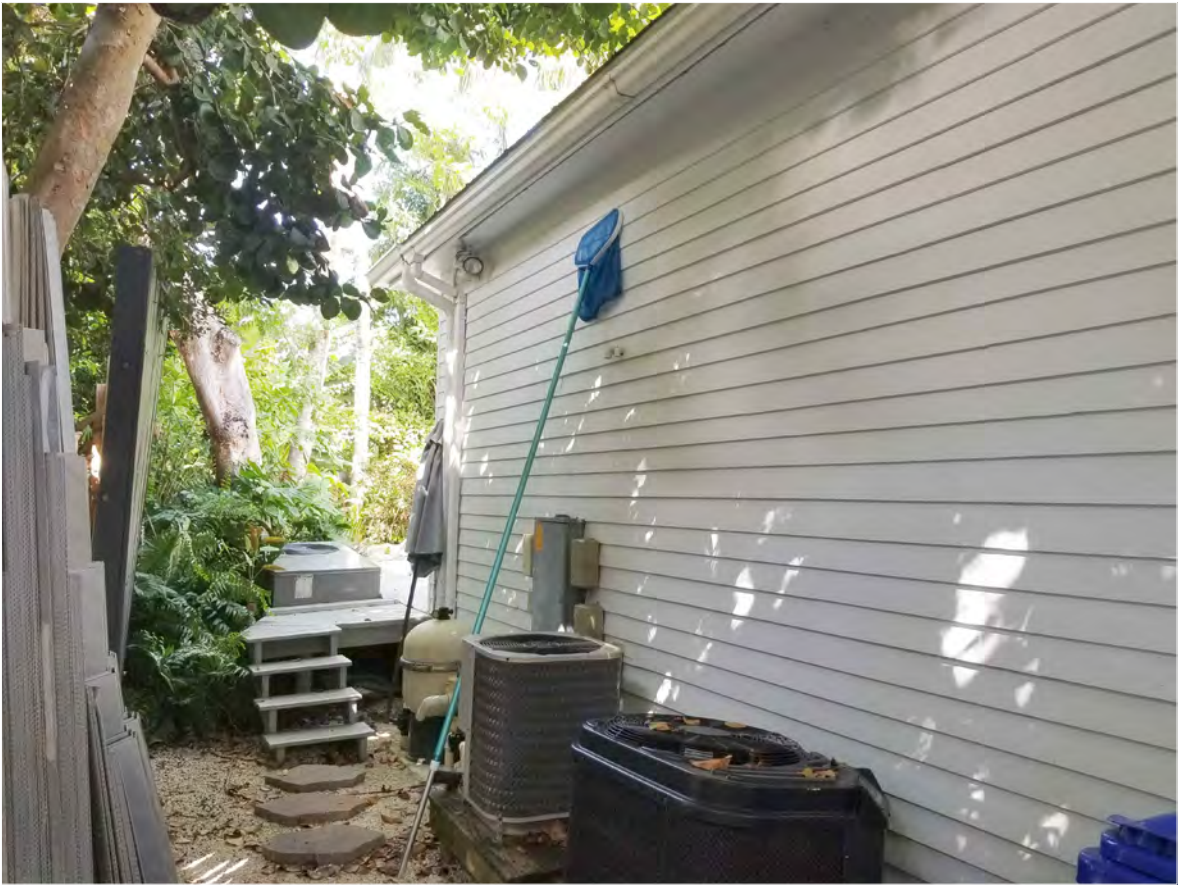
LEFT SIDE VIEW OF PRIMARY STRUCTURE
