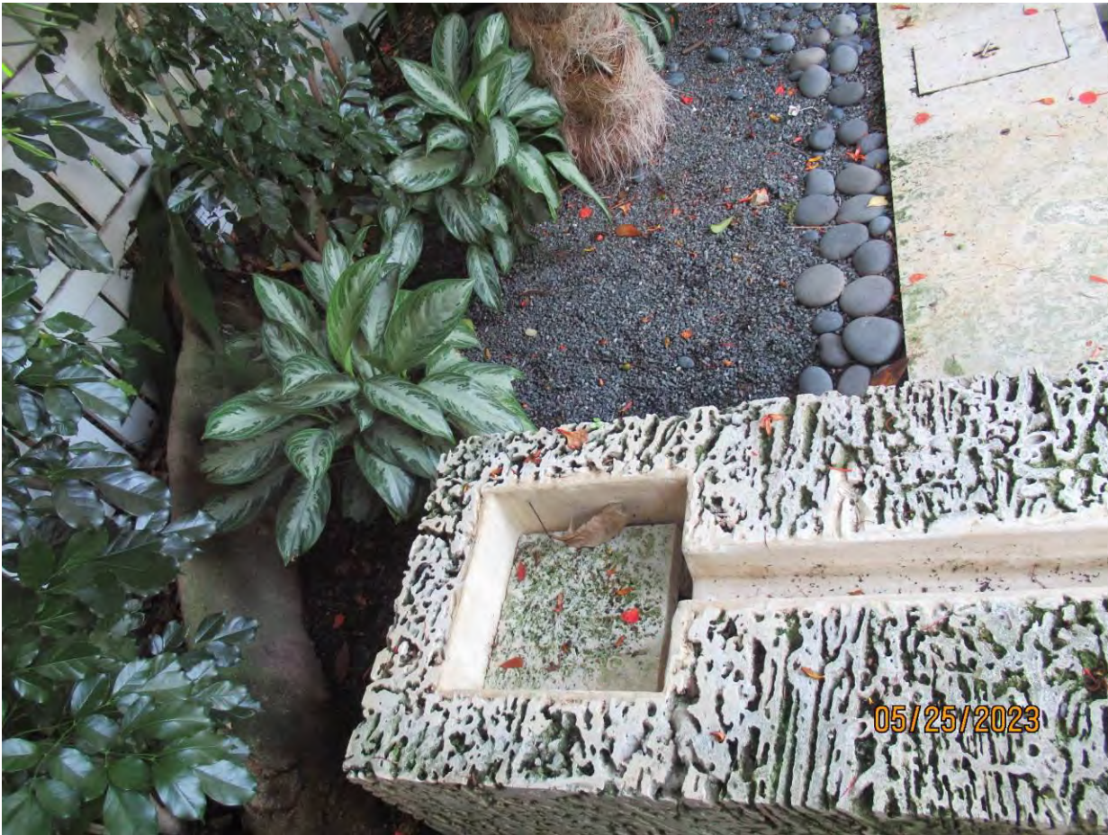
Photo taken from neighbor's property of roots from Royal Poinciana tree, view 3.
