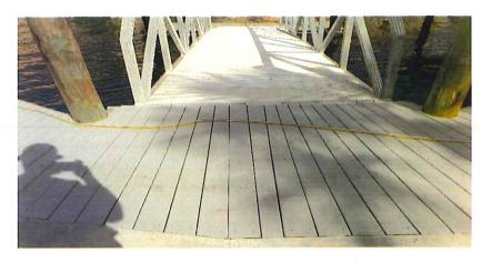
water lines, new dedicated fire line, DDCV backflow preventer and new fire cabinets. A new addition to the marina was the installation of a composite decked floating dock with 12" solid composite dock piling and an aluminum access gangway. Clean fill was brought in to raise the grade to meet the new cap elevation for the owners' final landscaping plan.
