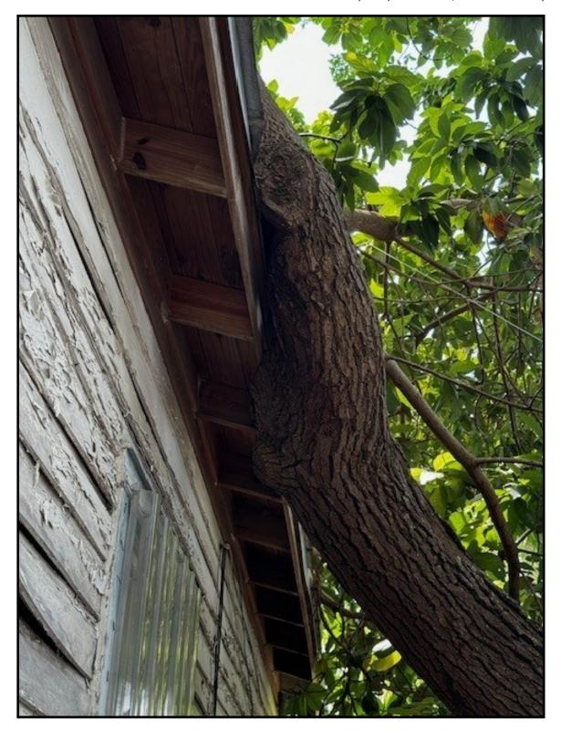
As you can see the trunk has damaged the roofline and soffit
