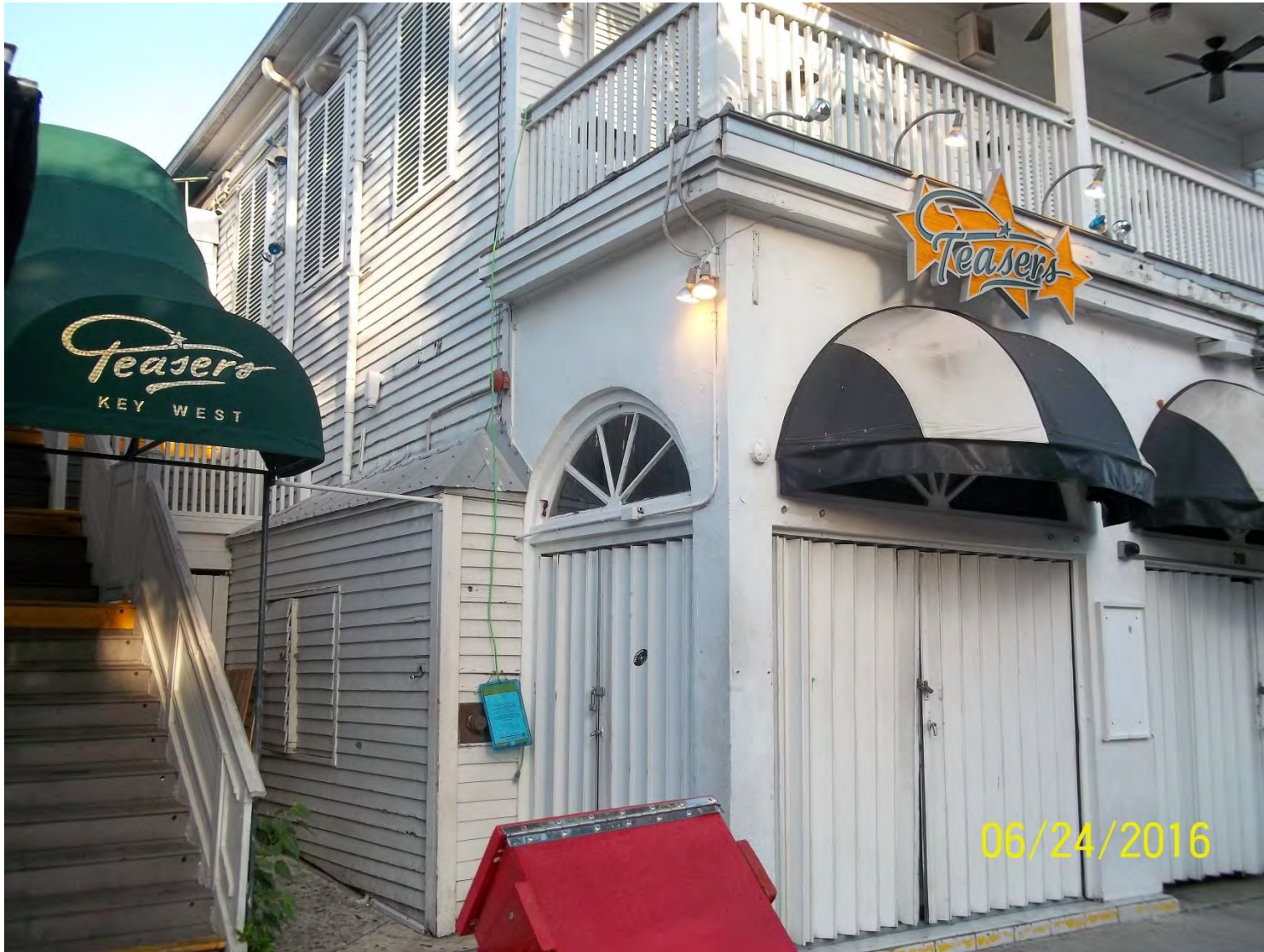
Last approved signs for the business – Photograph taken by Code Compliance before implementation of New Signage Ordinance.
