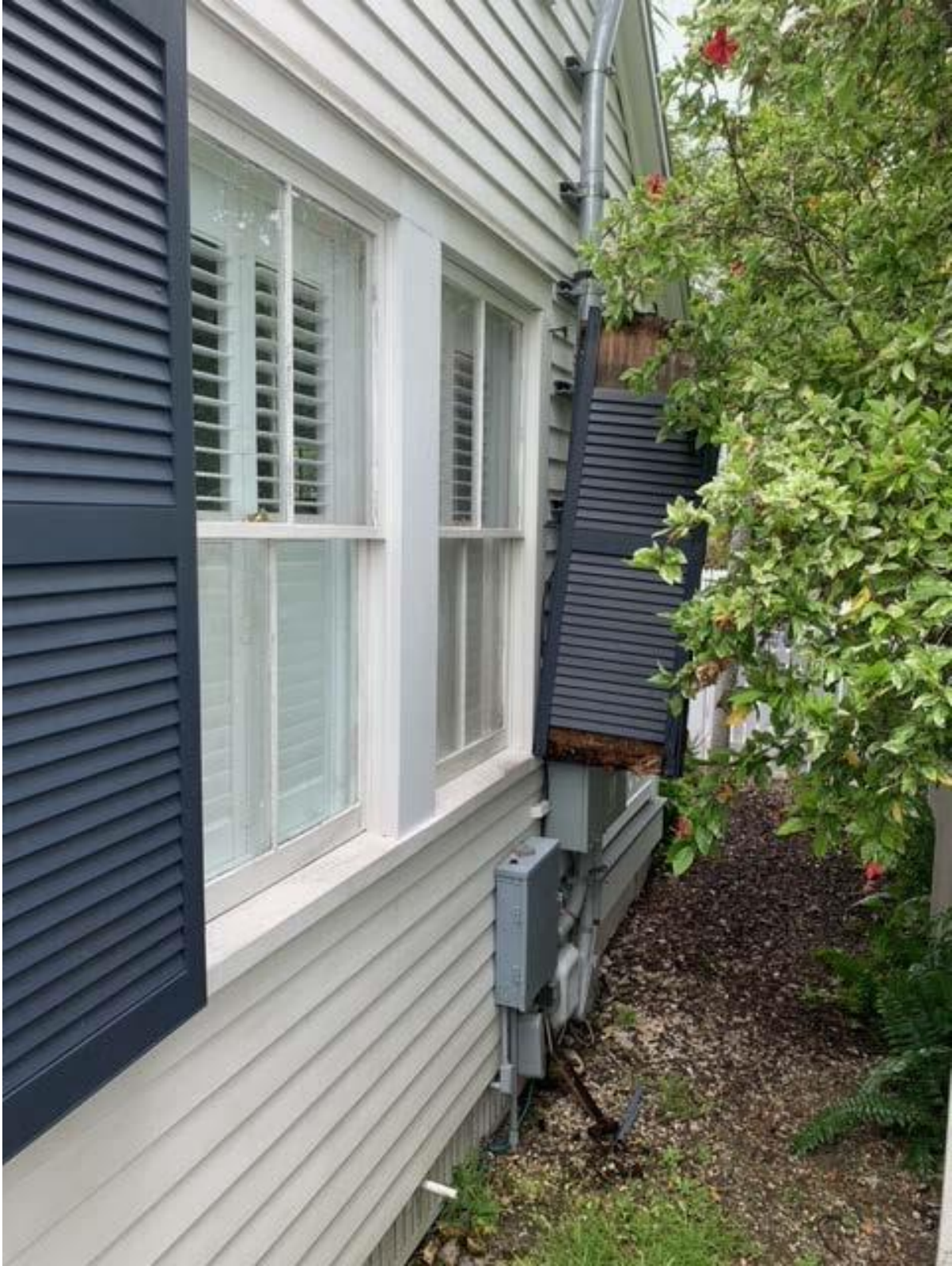
View of windows on East elevation of 1012 Southard Street.
