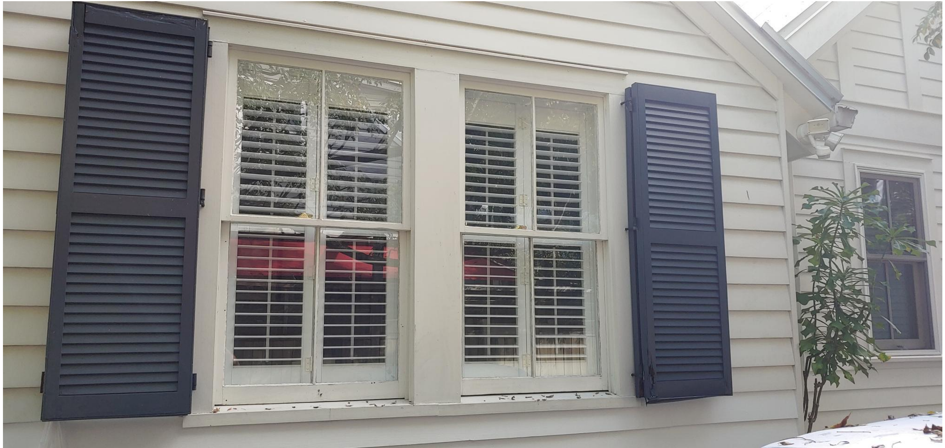
Windows on West Elevation. 1012 Southard Street. Photo by Brandon Celli.
