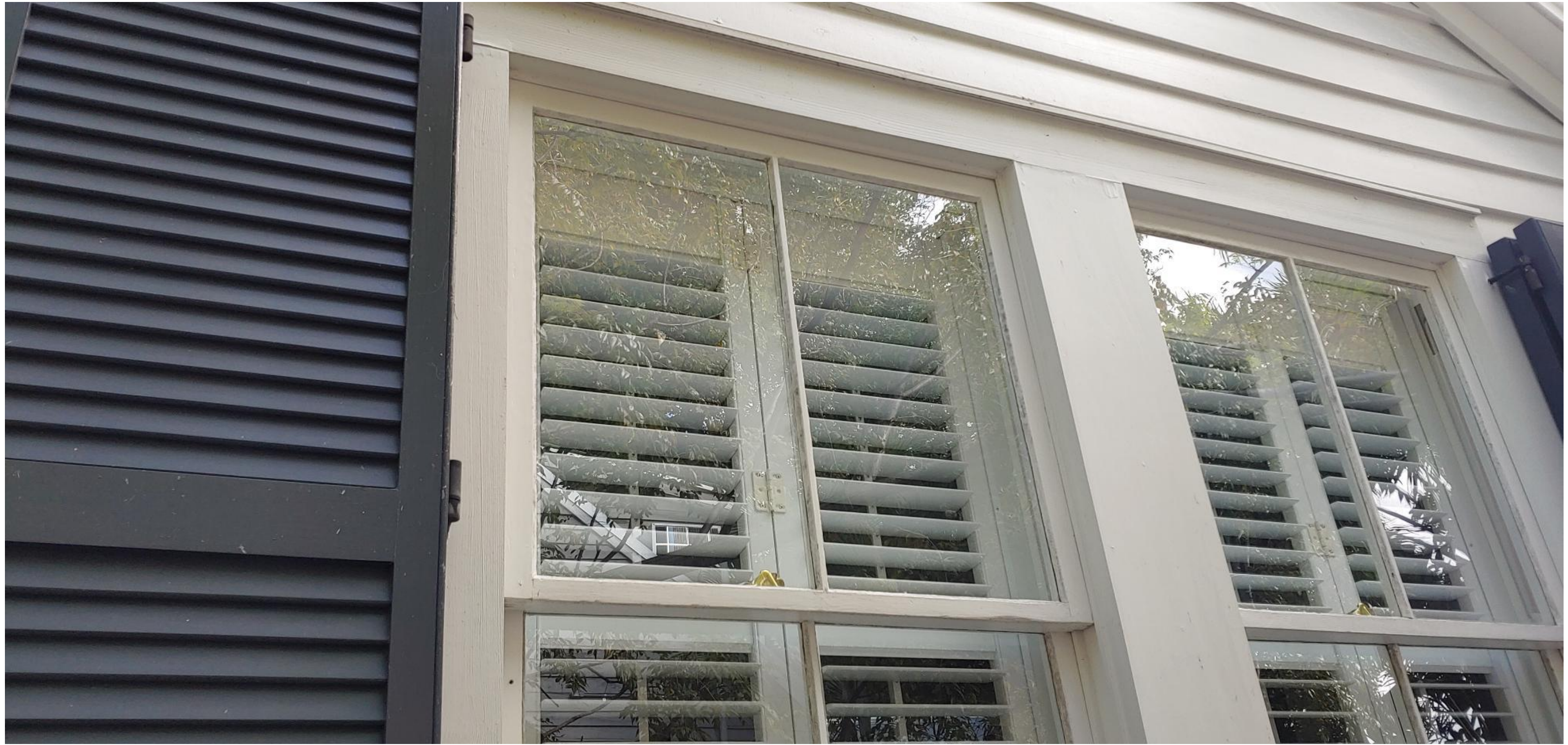
Windows on West Elevation 2. 1012 Southard Street. Photo by Brandon Celli.
