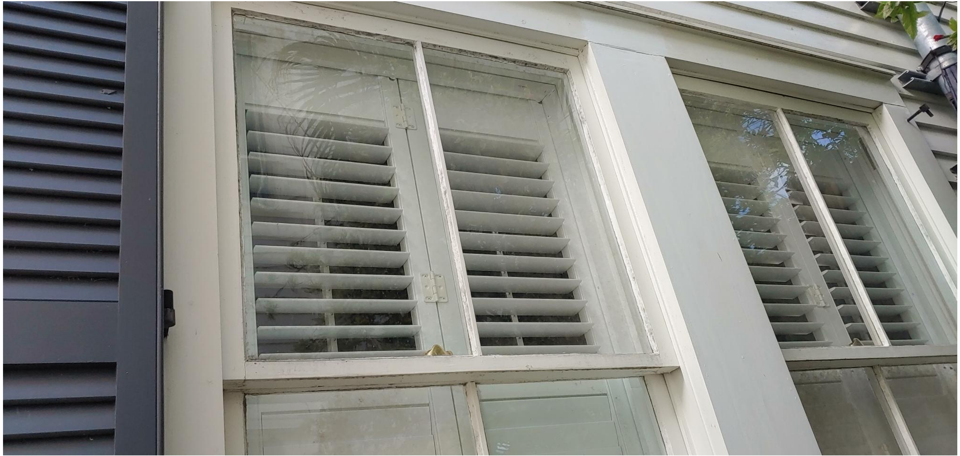
Windows on East Elevation. 1012 Southard Street. Photo by Brandon Celli.
