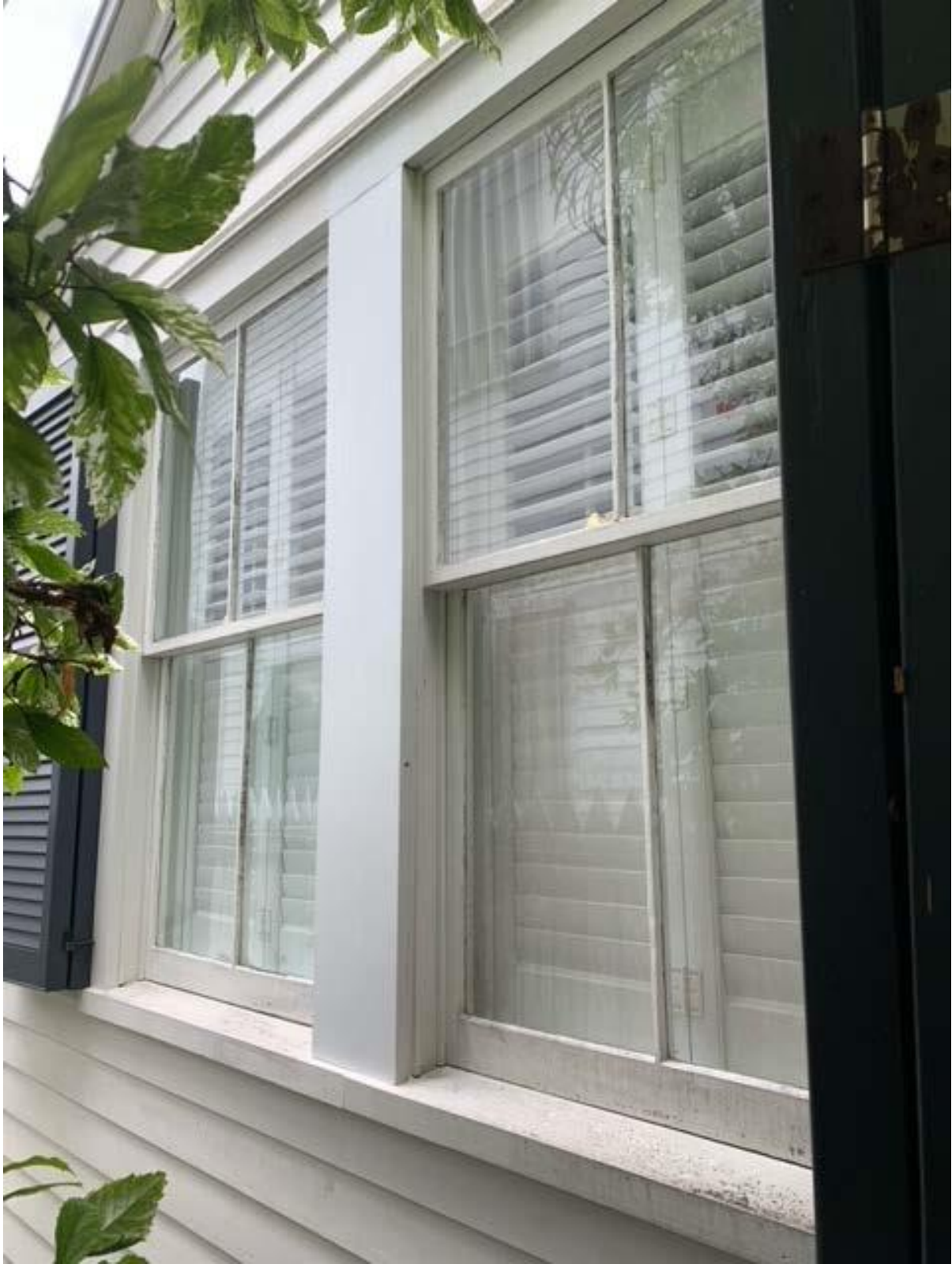
View 2 of windows on East elevation of 1012 Southard Street.
