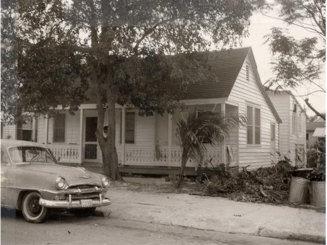
1965 photo showing the house at 1012 Southard Street.
