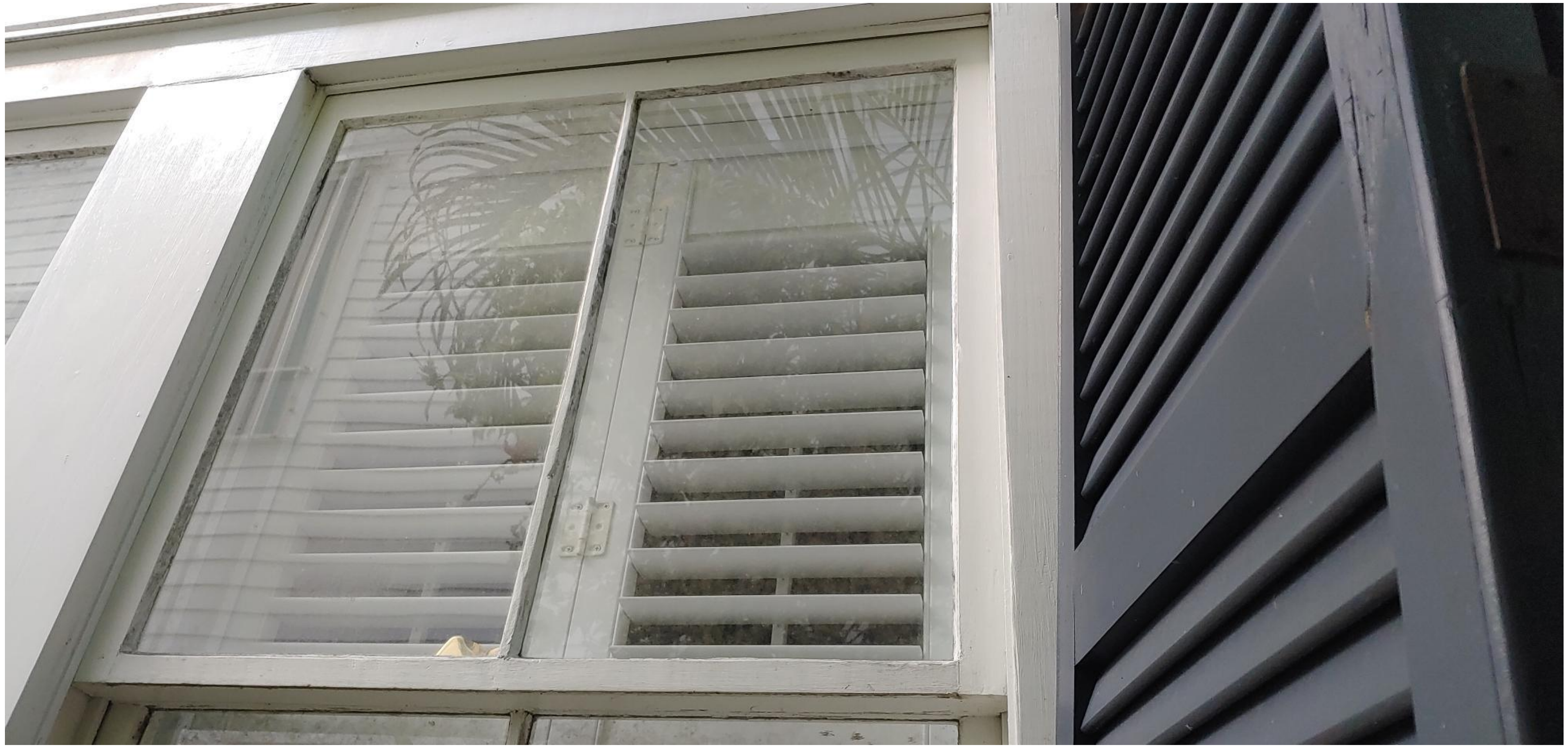
Up-close Window on East Elevation. 1012 Southard Street. Photo by Brandon Celli.
