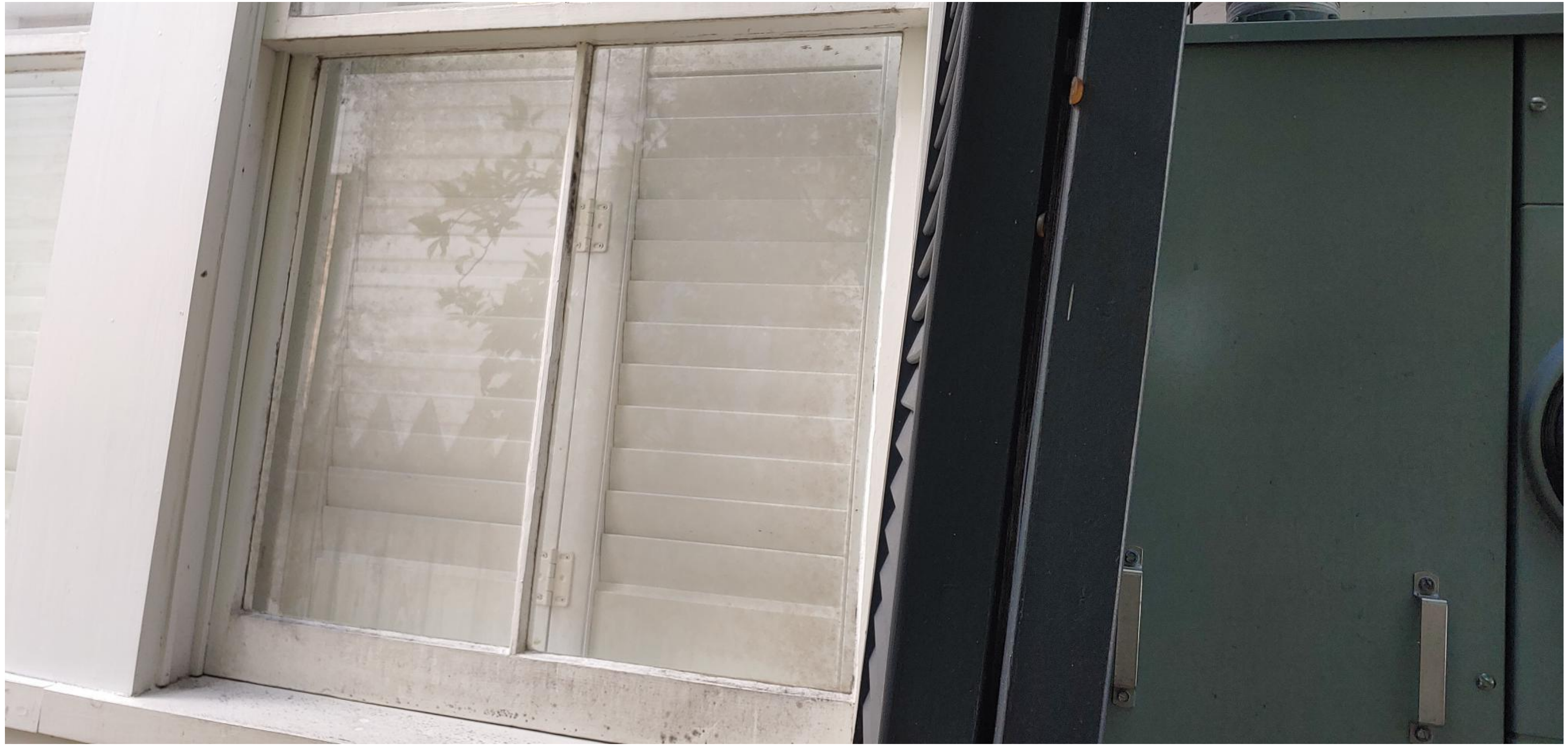
Up-close Window on East Elevation 2. 1012 Southard Street. Photo by Brandon Celli.
