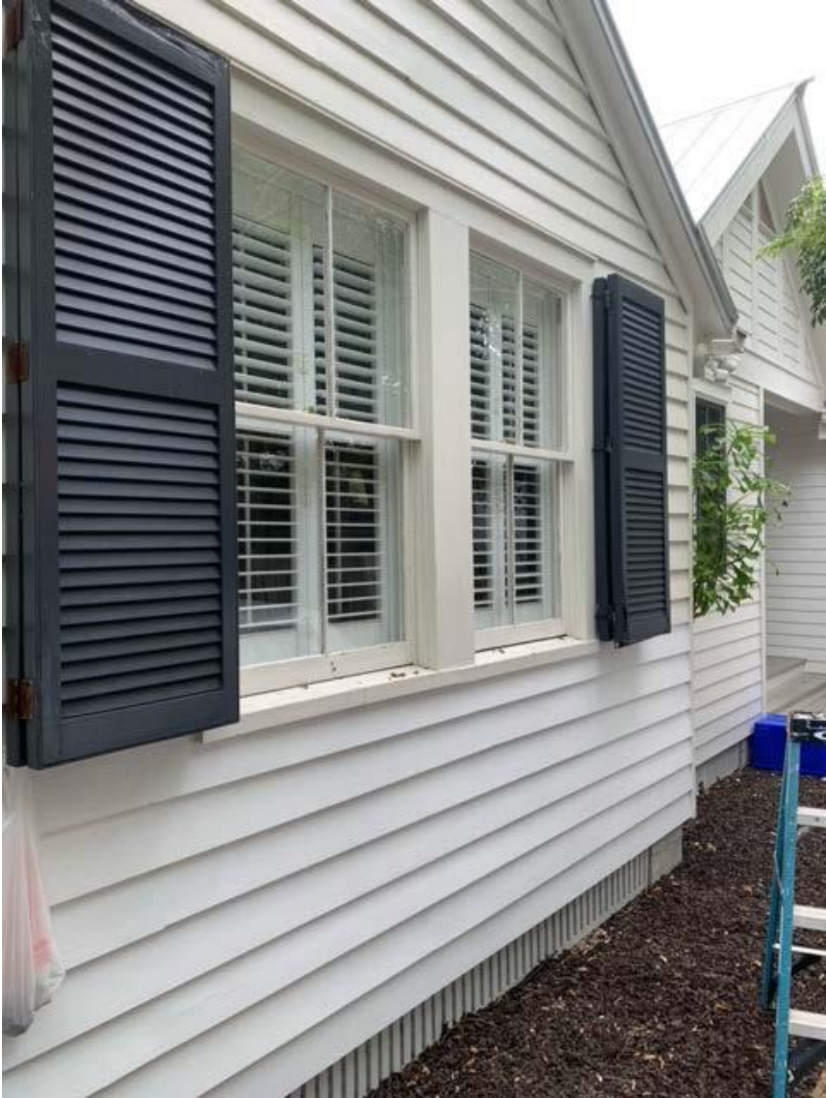
View of windows on West elevation of 1012 Southard Street.
