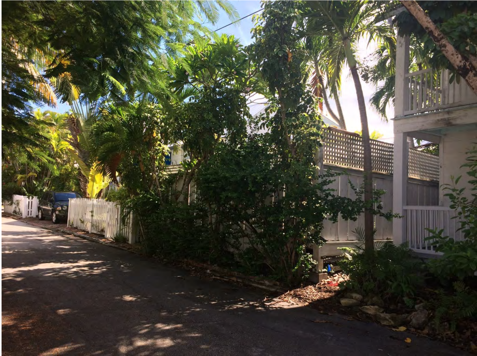
713 Eaton Street LEFT NEIGHBORING PROPERTY FRONT VIEW
