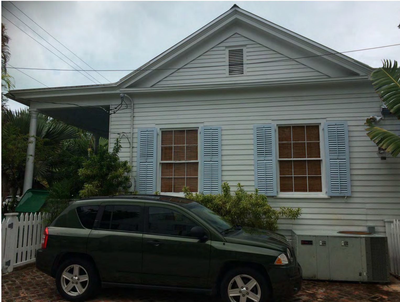
713 Eaton Street LEFT NEIGHBORING PROPERTY FRONT VIEW
