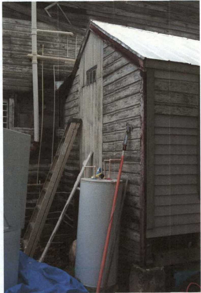
REAR FACADE + ADDITION
