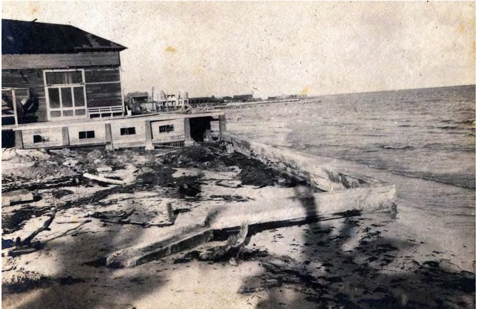
Historic Athletic Club at the end of Duval Street after the hurricane of September 1919.
