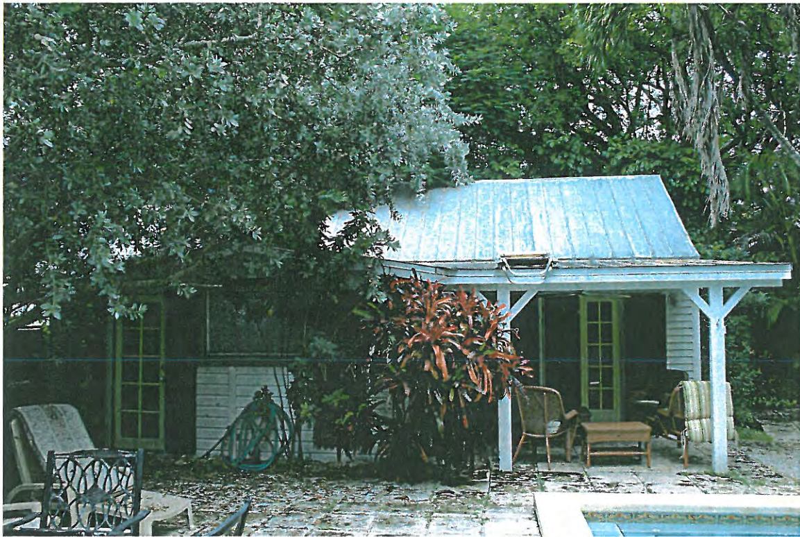
ROOF REPLACEMENT - REMOVE PATIO SHED ROOF & COLUMNS.
