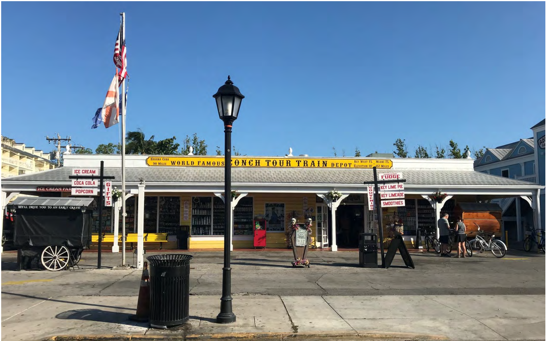
501 FRONT STREET FRONT VIEW
