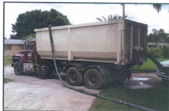
Sealed Truck Collects Dredge Material
