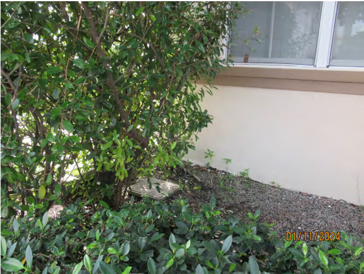
Photo of building corner-no cracks or roots observed.
