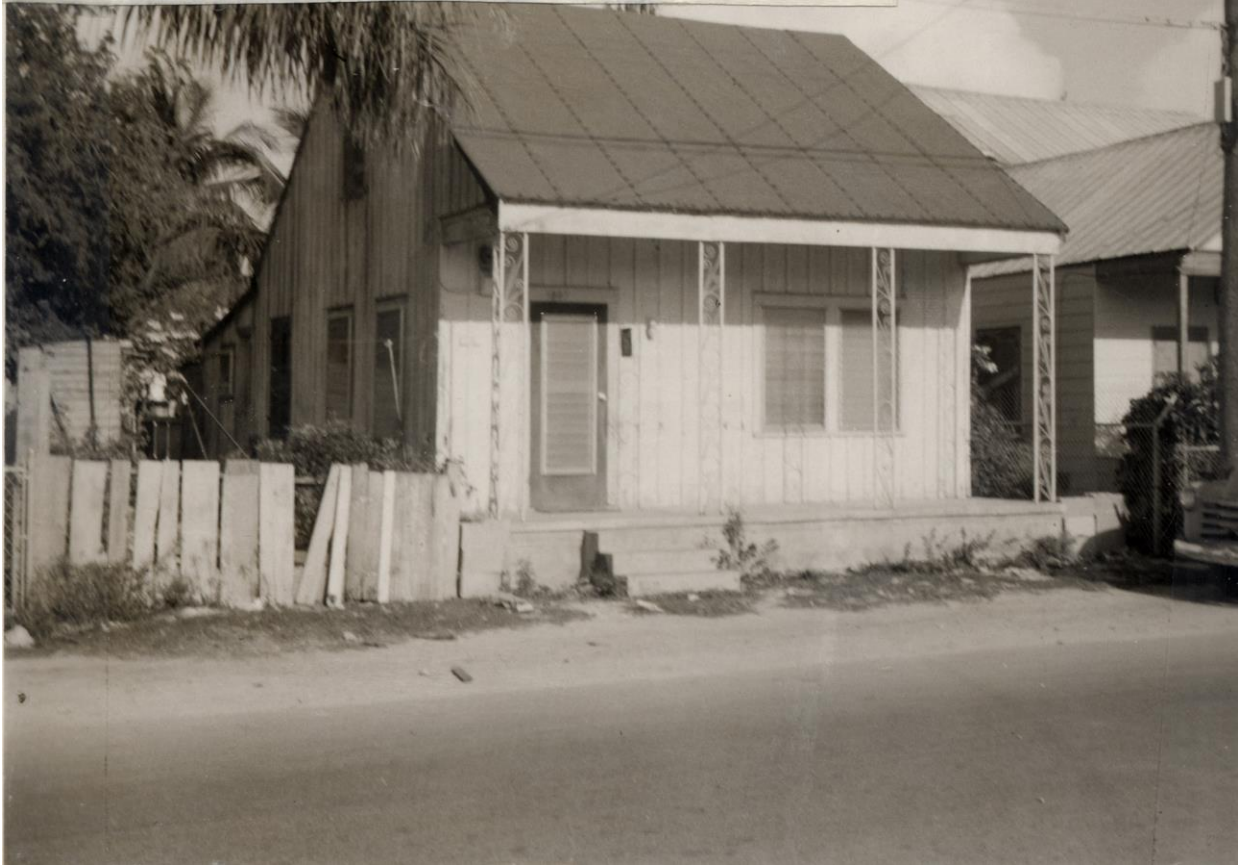
1965 photo of the structure at 1007 Thomas Street. Monroe County Public Library's record provides a year built ca. 1918.
