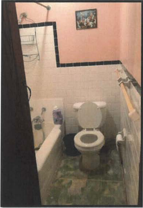
Unit 9 Lockout – bathroom
