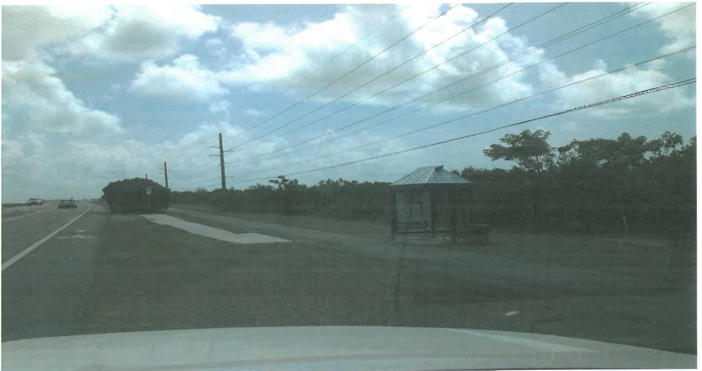
ADA Ramp - Baypoint
