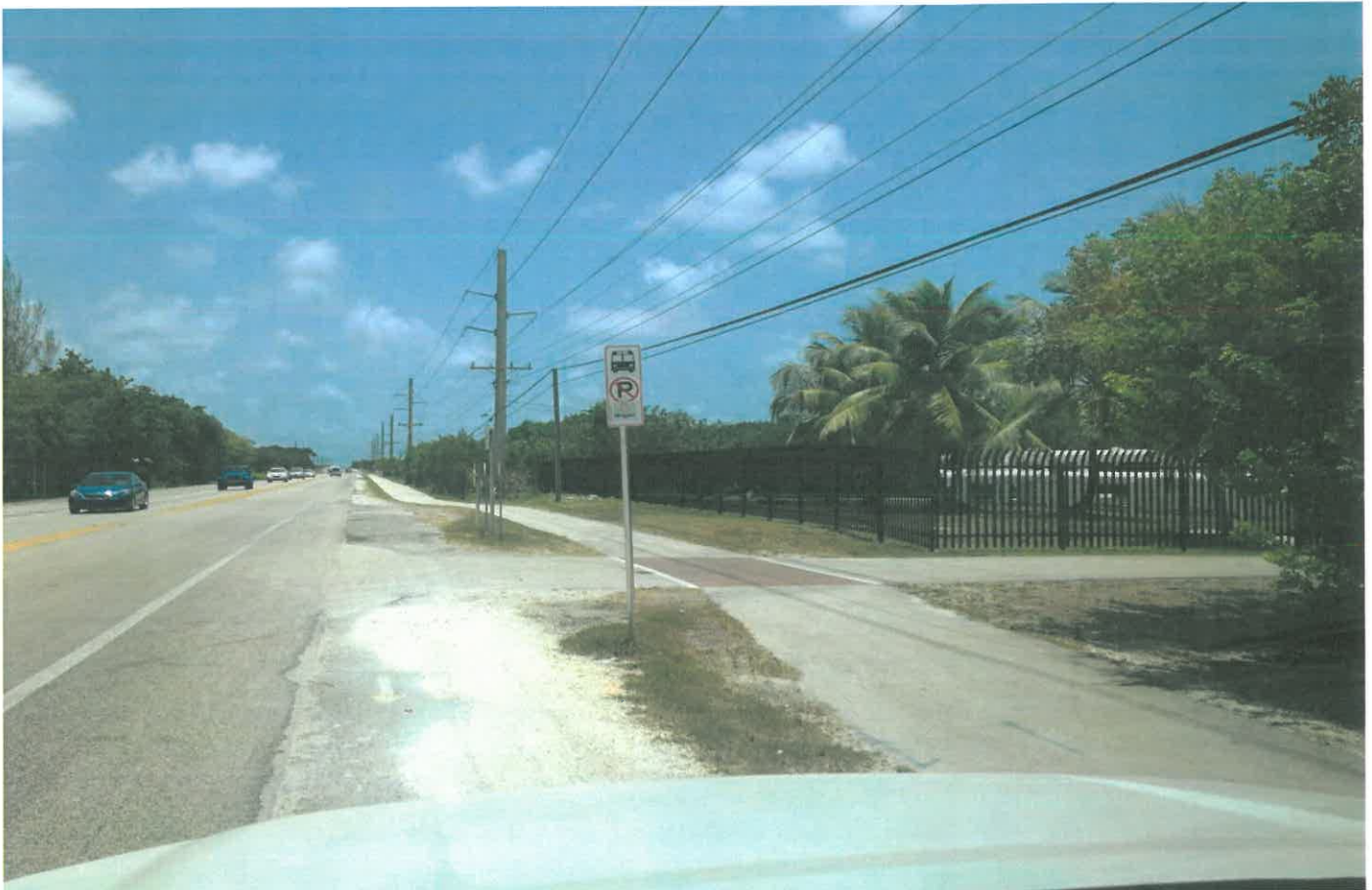
FKAA Pump Station - Ramrod
