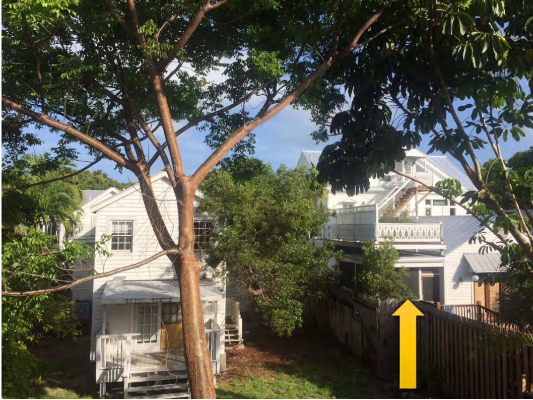
REAR OF PROPERTY AND REAR OF NEIGHBOR TO WEST
