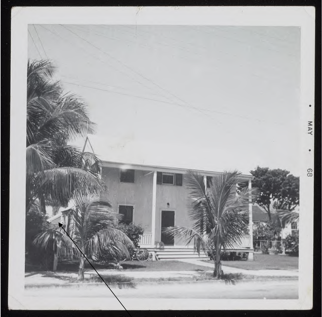
This is a 1938 photo of the house (the May 1968 date is incorrect) The outbuilding in the rear of the property can be seen to the left of the house. This is the proposed location of the ADA restroom.
