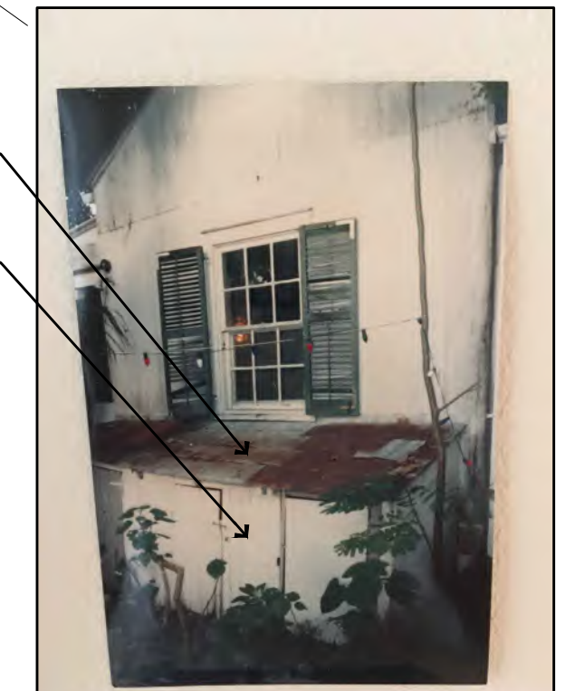
THIS PHOTO SHOWS THE HISTORIC SHED FOR THE PUMPS. THIS SHED SHALL BE REBUILT IN THIS CONFIGURATION.
