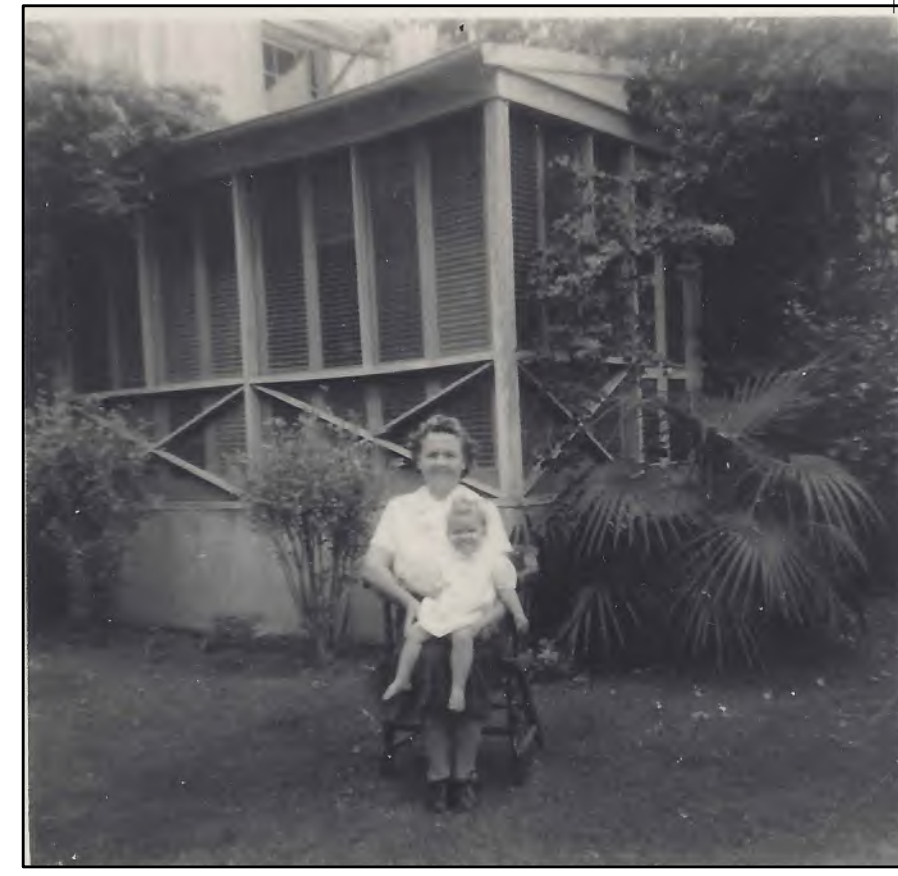
THIS 1950s PHOTO SHOWS THE ORIGINAL 1941 CISTERN PORCH. THE PORCH SHOULD BE RESTORED TO THIS CONFIGURATION.
