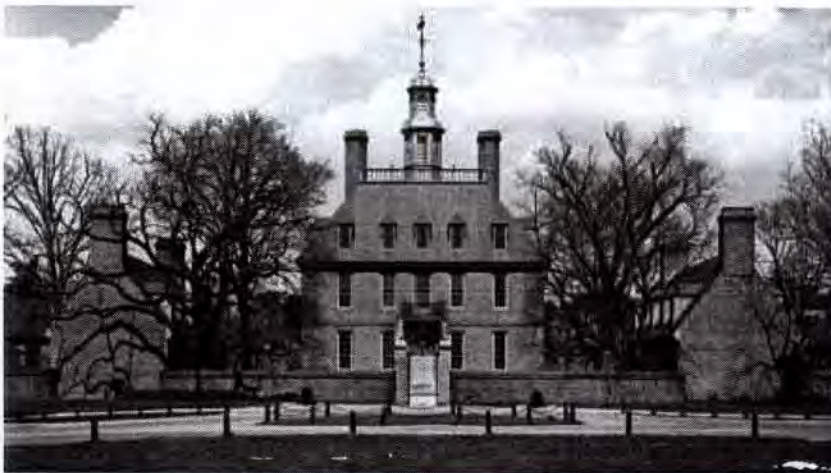
In the 1930s reconstruction of the 18th century Governor's Palace at Colonial Williamsburg, Virginia, the earliest archeological remains of the brick foundation were carefully preserved in situ, and serve as a base for the reconstructed walls. Photo: The Colonial Williamsburg Foundation.
