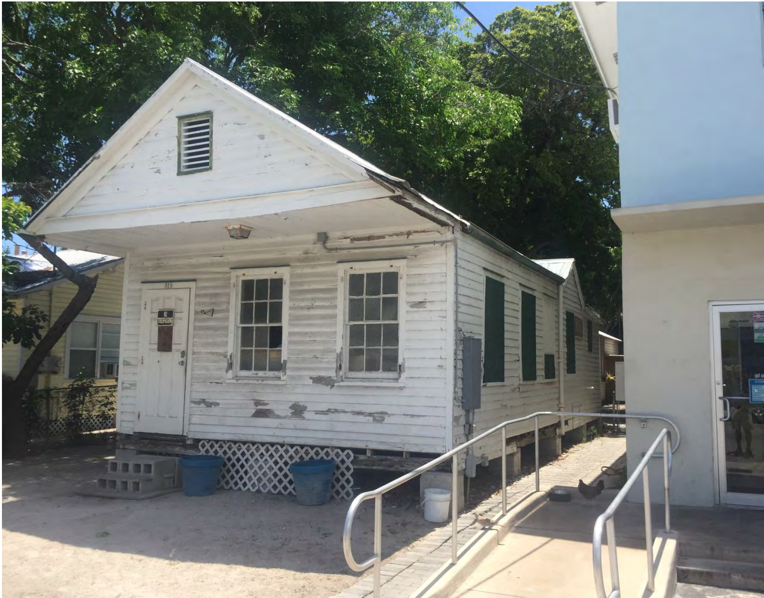
VIEW FROM WINDSOR LN.
