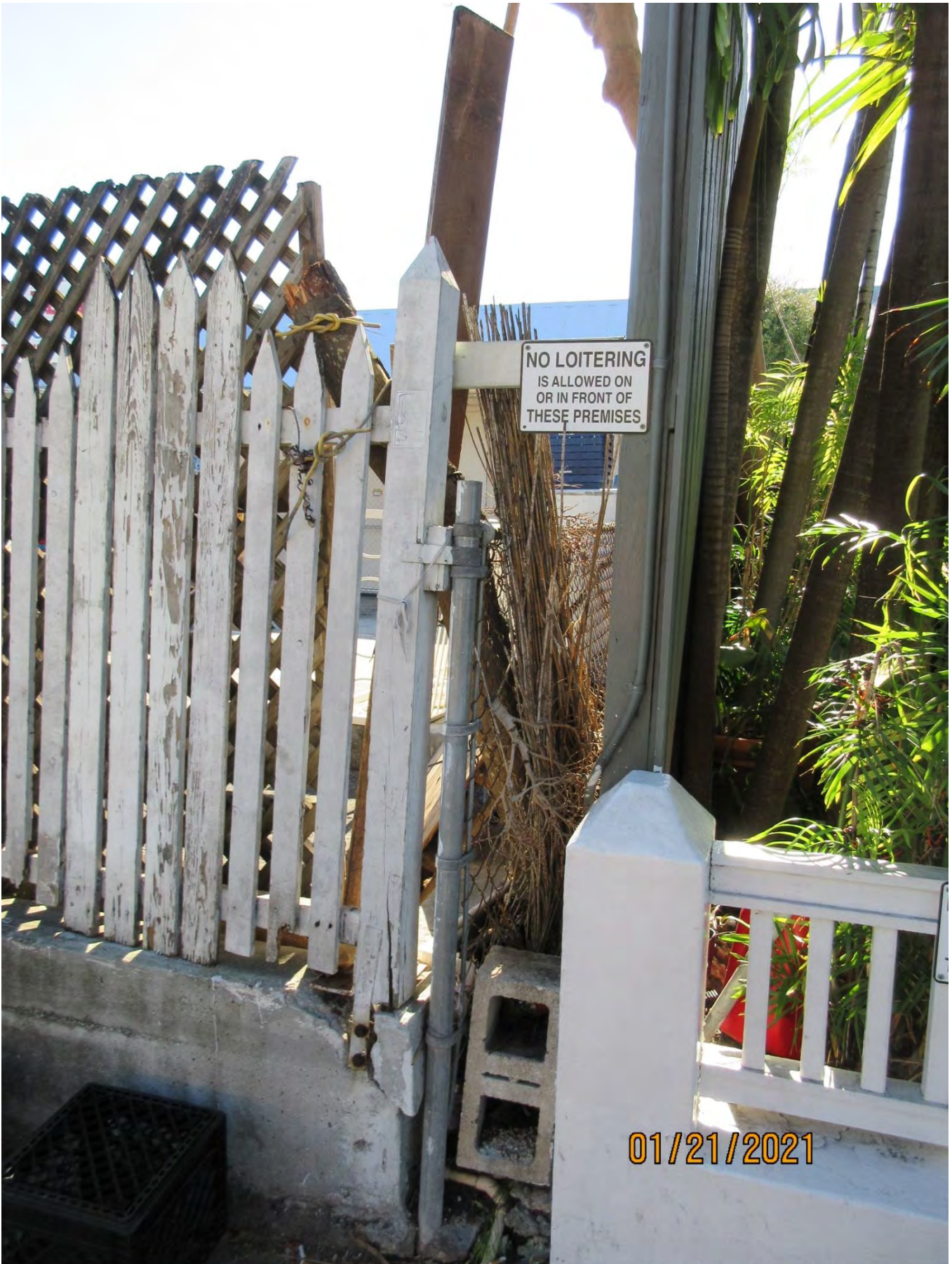
Photo looking at the property line on Fleming Street.
