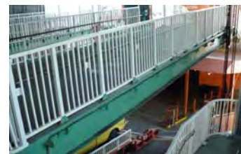
Moveable Transfer Bridges
