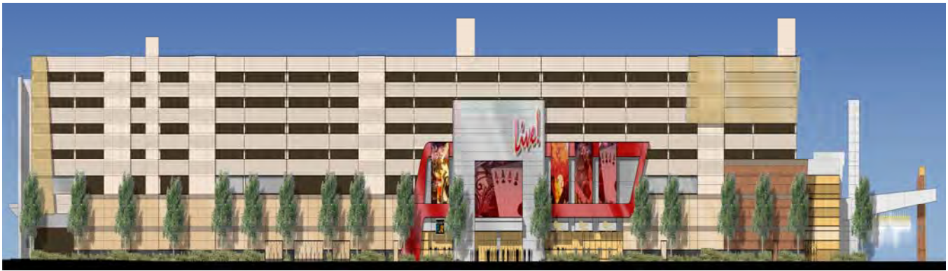
Maryland Live Casino – 1.7 Million SF Building Opened in 2012
