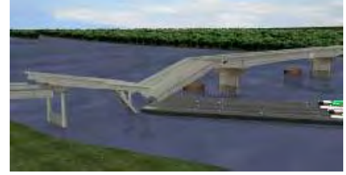
Video Analysis of Bridge Collapse
