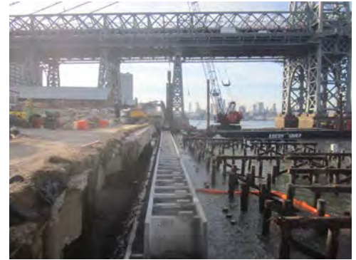
Precast Gravity Wall On-Top Existing Seawall Foundation
