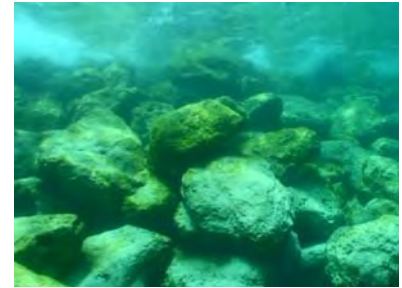
Hard Rock Hotel & Casino Punta Cana - Breakwater Dive Inspection
