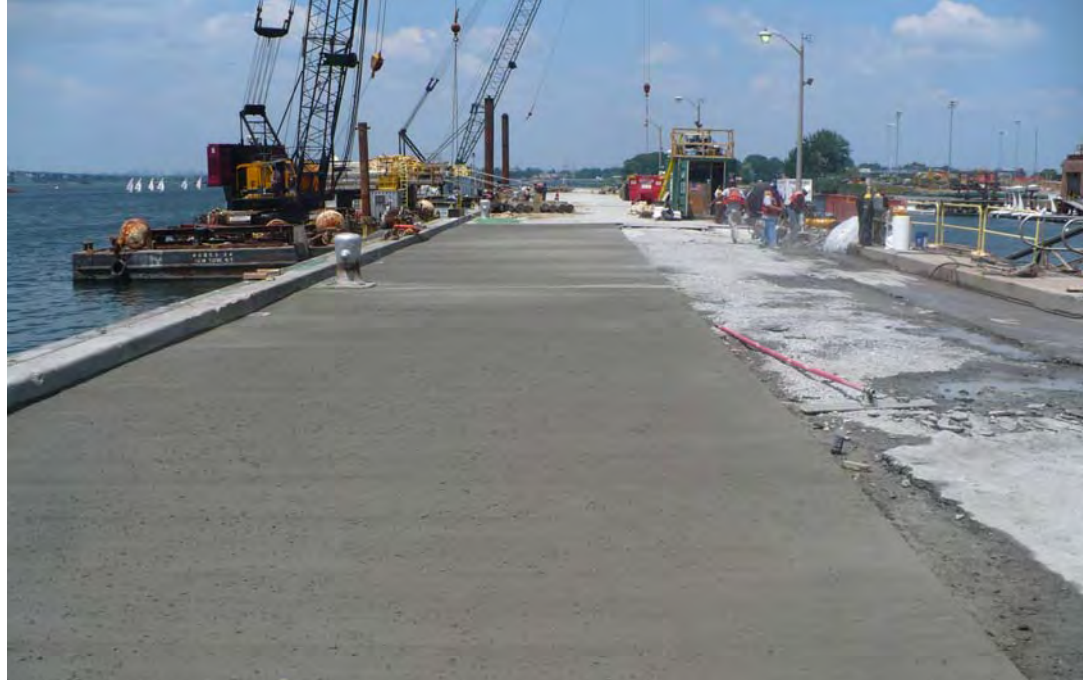
Pier Under Construction
