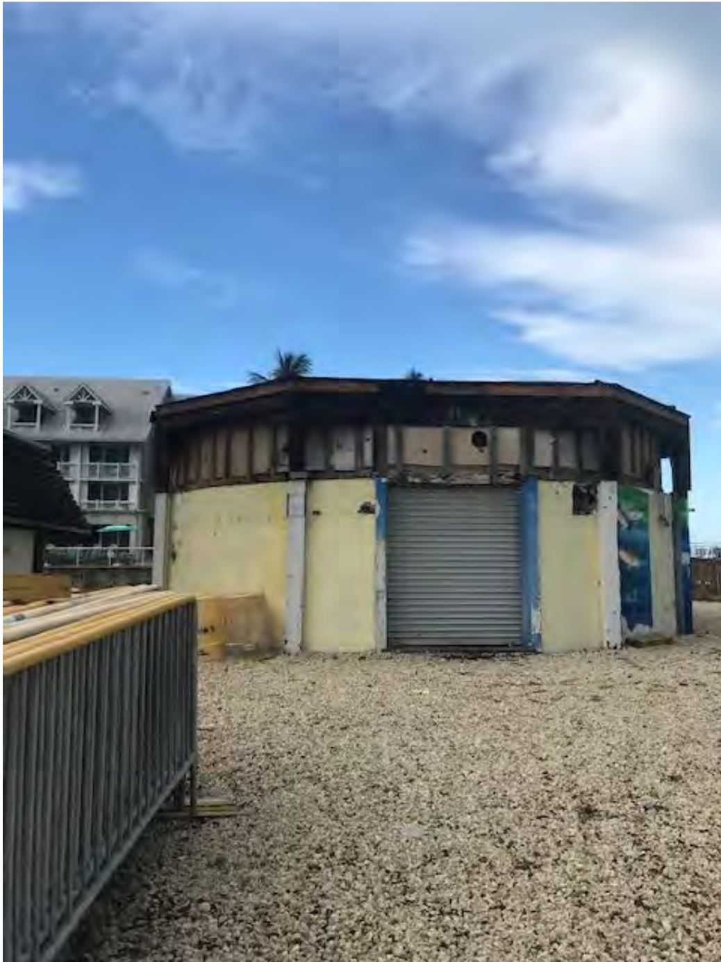
Photograph of westernmost Cable Hut from Mallory Square.
