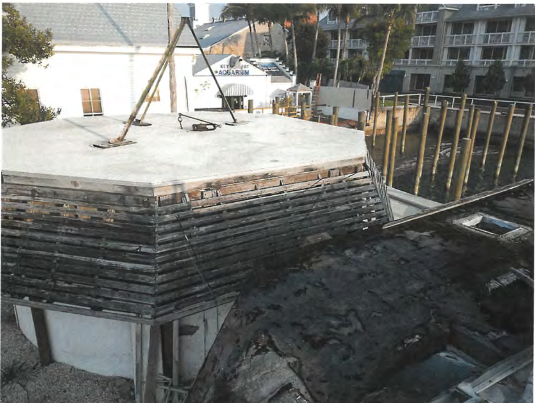
Roof of East Cable Hut.
