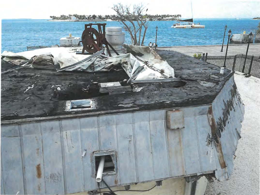
Roof of West Cable Hut.
