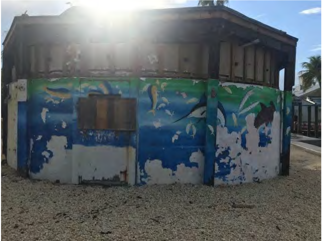
Westernmost Cable Hut photograph facing east.
