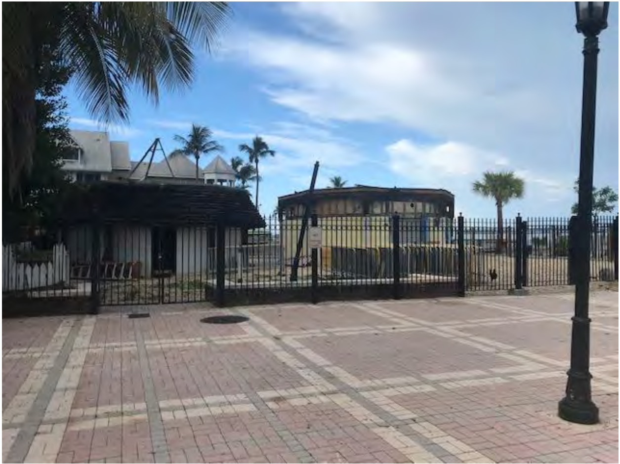
General view of both Cable Huts from Mallory Square.
