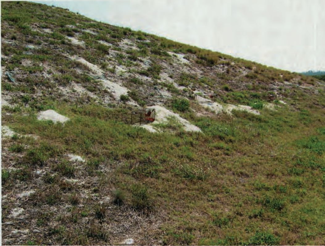
Stock Island Landfill – Southwest Face – View South
