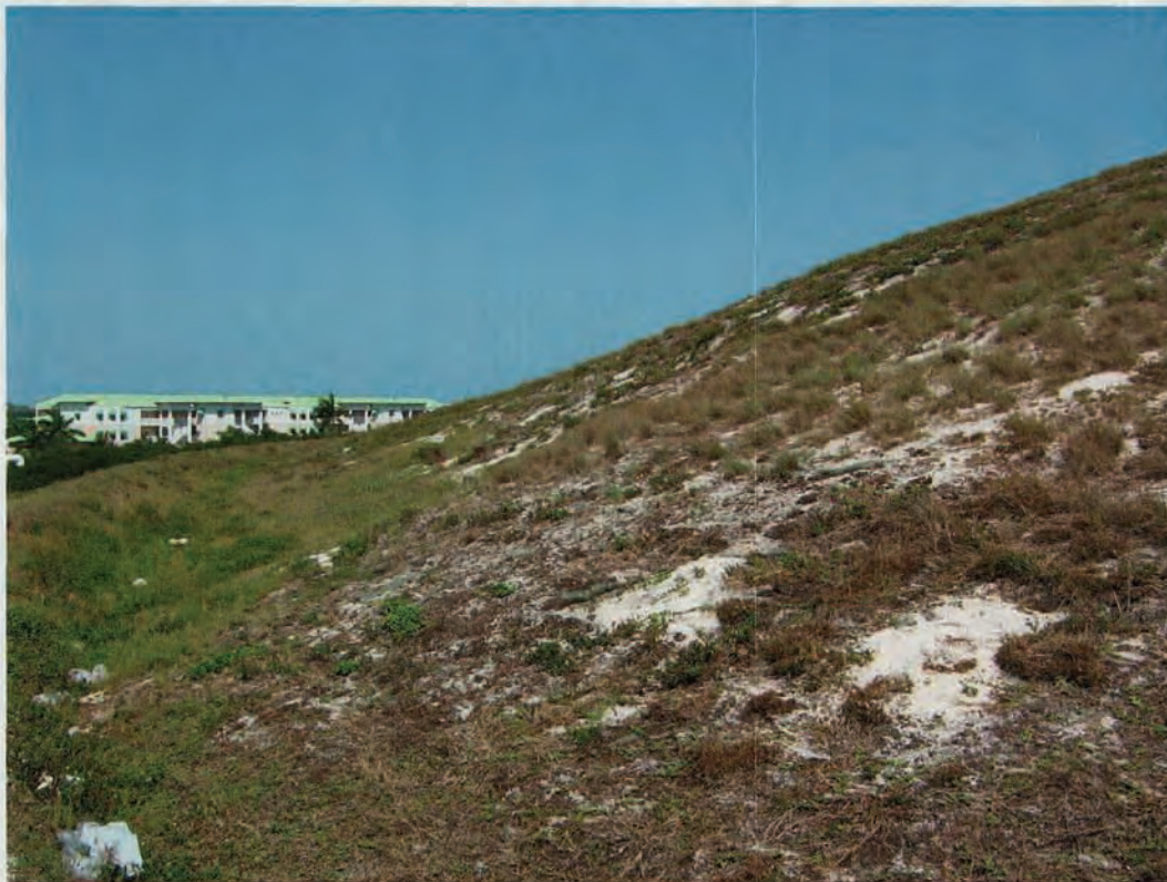
Stock Island Landfill – Southwest Face – View North
