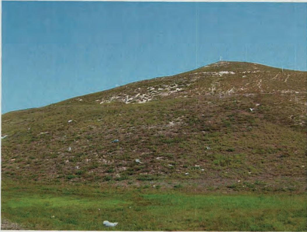
Stock Island Landfill – Southwest Face – View East
