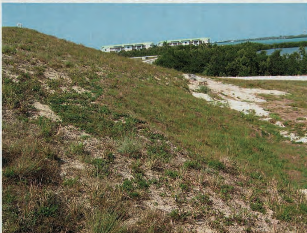
Stock Island Landfill – North Face – View West
