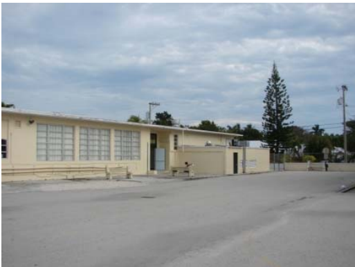
Building C – Picture 5
