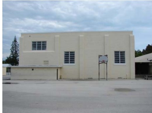
Building D – Picture 4
