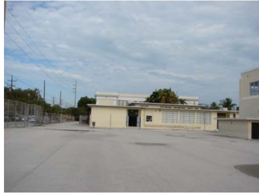
Building C – Picture 2
