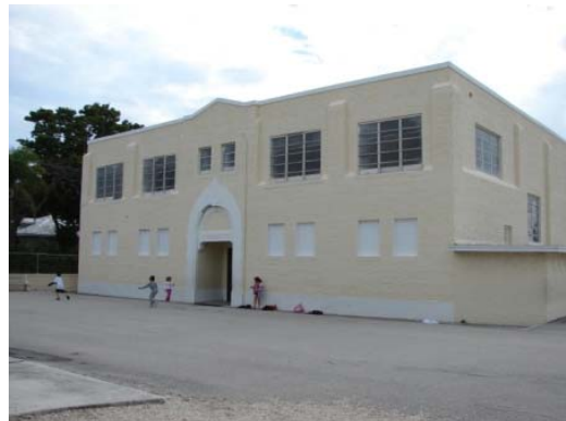
Building D – Picture 6
