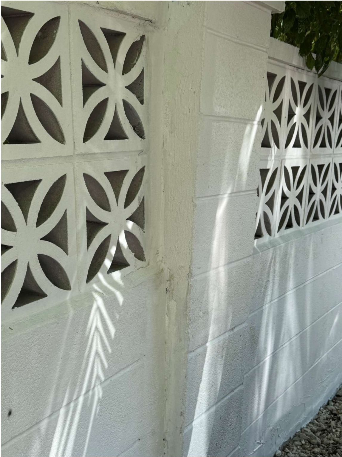
Tree's roots have caused significant structural damage to the concrete wall.
