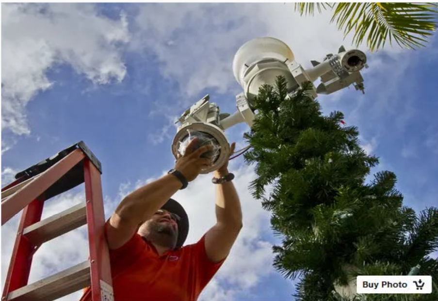
Tomas Duran, a technician with Integrated Fire and Security Solutions, install one of the surveillance cameras on First Street in Downtown Fort Myers, Wednesday afternoon (12/23/15). (Photo: Ricardo Rolon / The News-Press)
