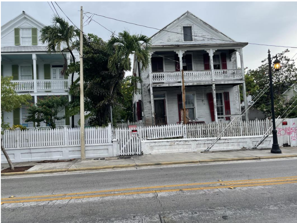
Close View of adjacent Northern Property
