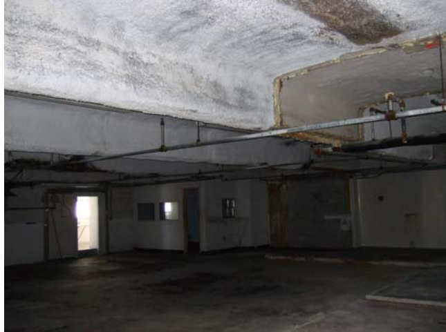
Photo 05 - Building Structure C First Floor
