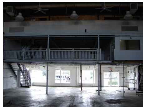
Photo 04 Building Structure B Second and Third Floor Terraces
