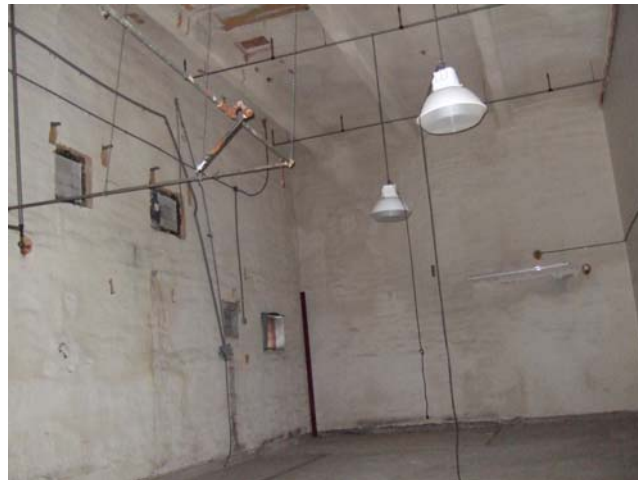
Photo 06 - Building Structure D First Floor
