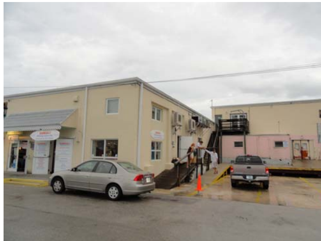
Photo 01- Building Structure A Two Story (West End)
