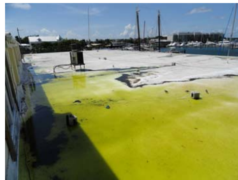
Photo 08 - Building Structure A Roof Coverings (Building Connection)
