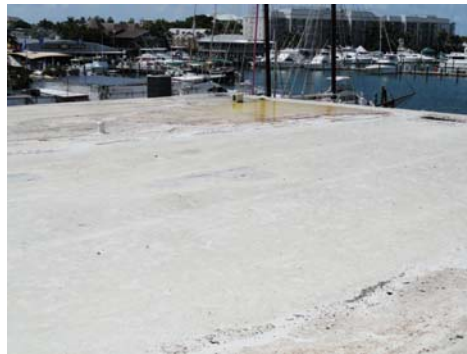
Photo 07 - Building Structure A Roof Coverings (West End)
