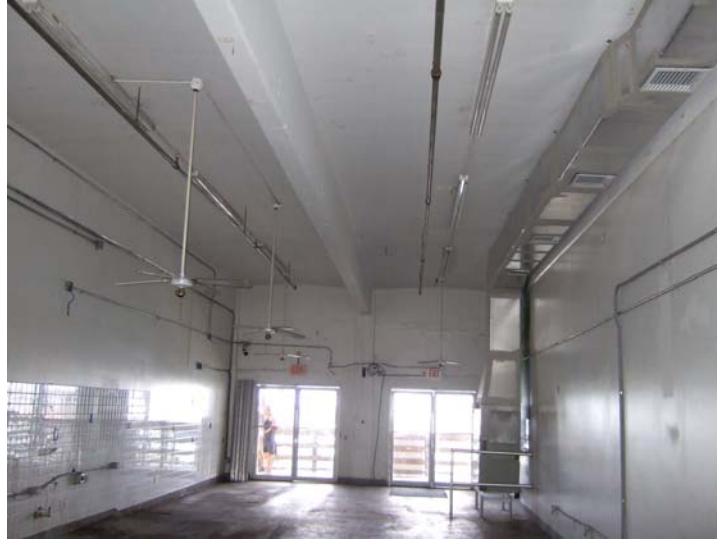
Photo 02 - Building Structure A One Story
