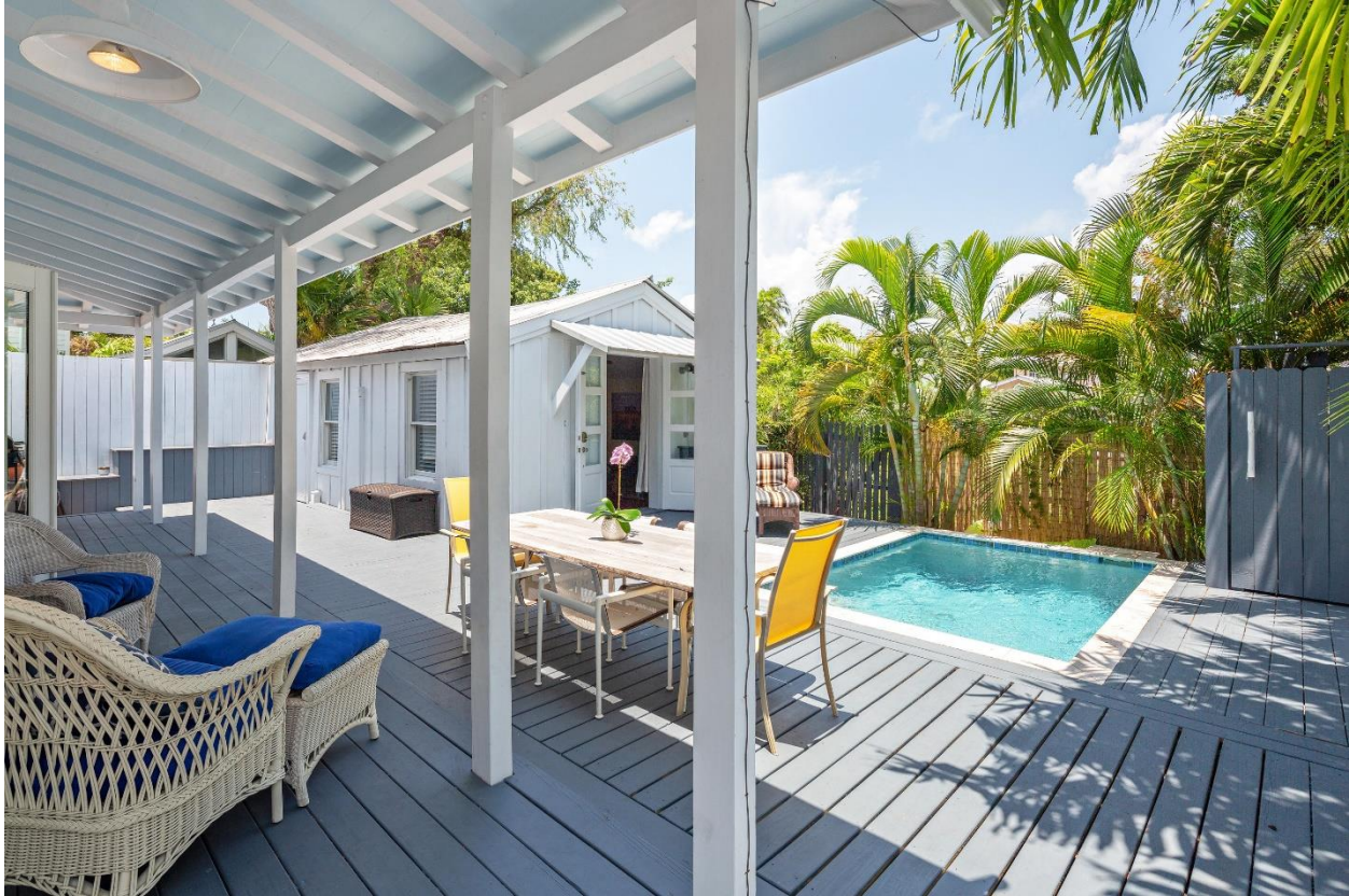
View of accessory structure.
