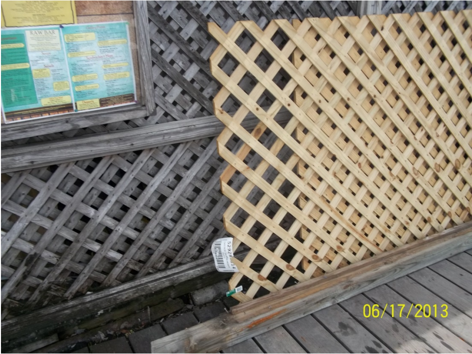
Schooner Wharf new lattice stored on the dock side of the bar next to unpermitted work.
