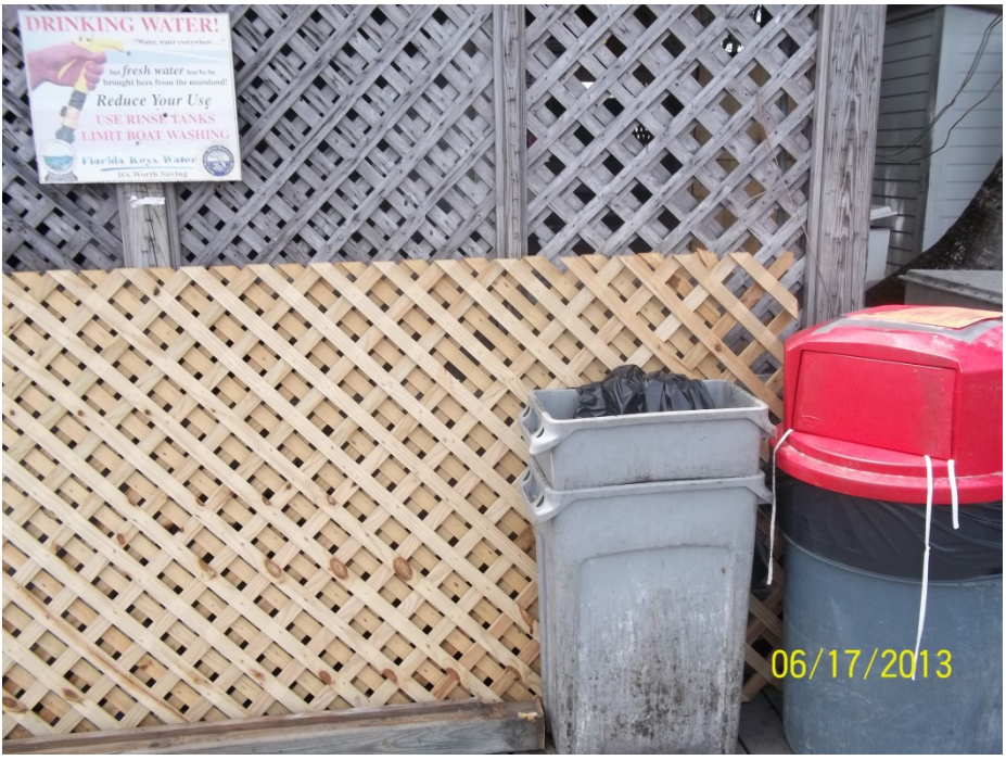
More Lattice work being stored next to unpermitted work
