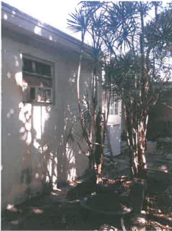
4. Photograph of the rear of the structure
