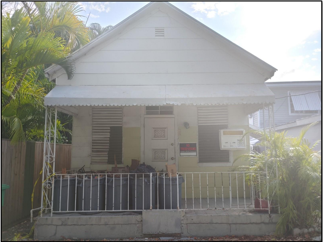
4 Havana Avenue – Site visit May 3, 2021
