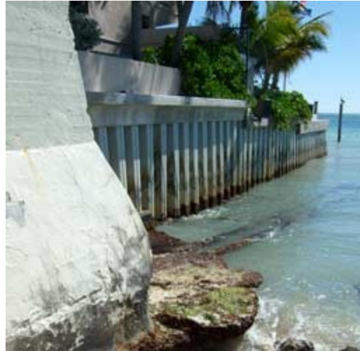
Detail of shore-end cables Photo: Bill Burns
