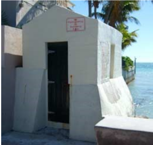
1917 cable hut, January 2010 Photo: Bill Burns
