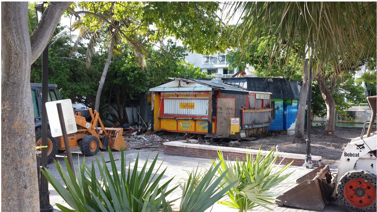
City Crew demolishing restaurant. October 5, 2013. Westin Resort prominent over the top.
