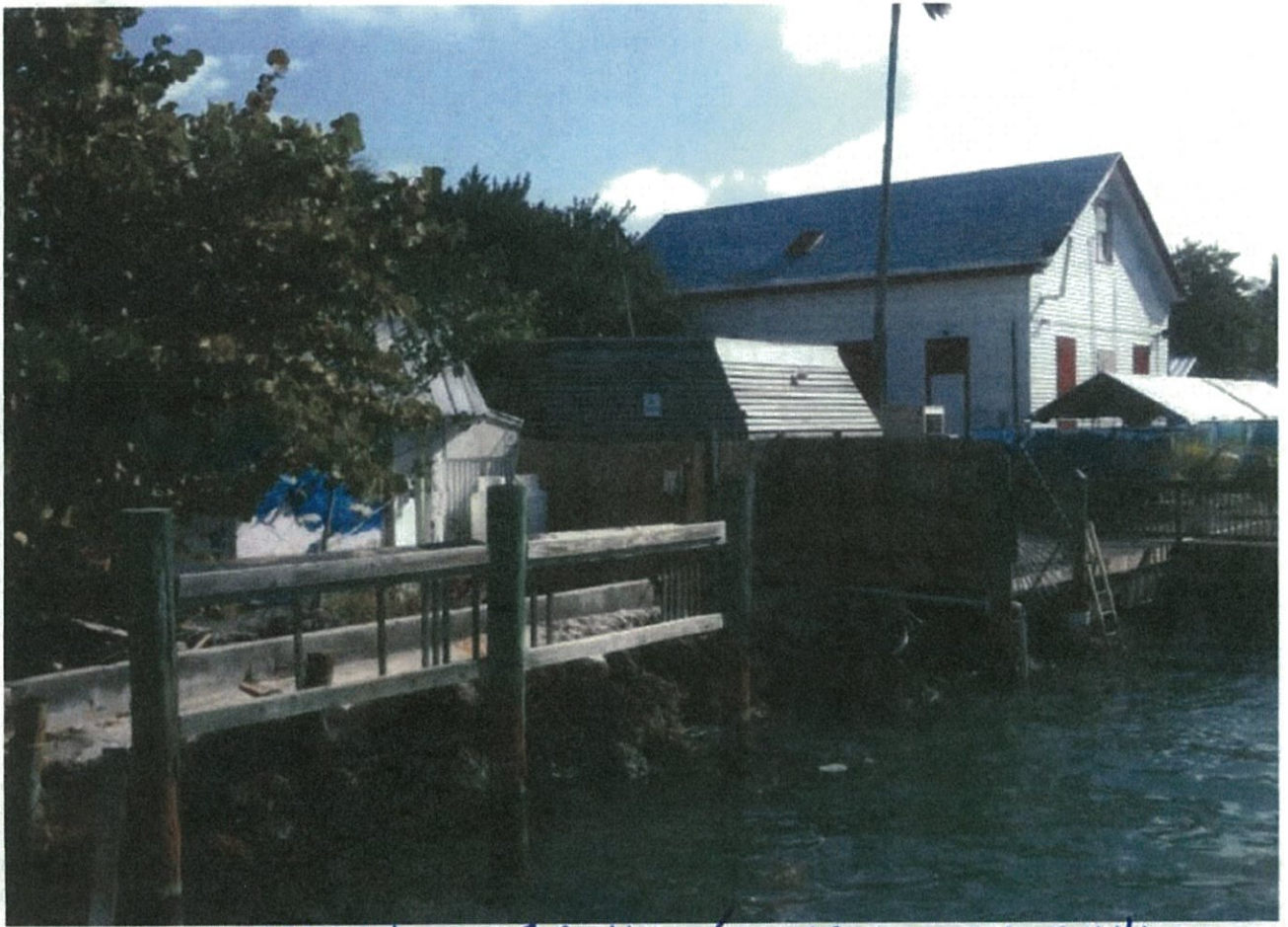
EXISTING BROKEN/ROTTED DECK BEHIND CISTERN
