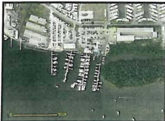
2008 aerial of marina post construction.
