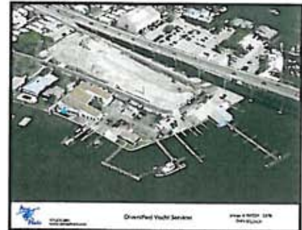
Aero Photo showing construction start with clearing of upland.
