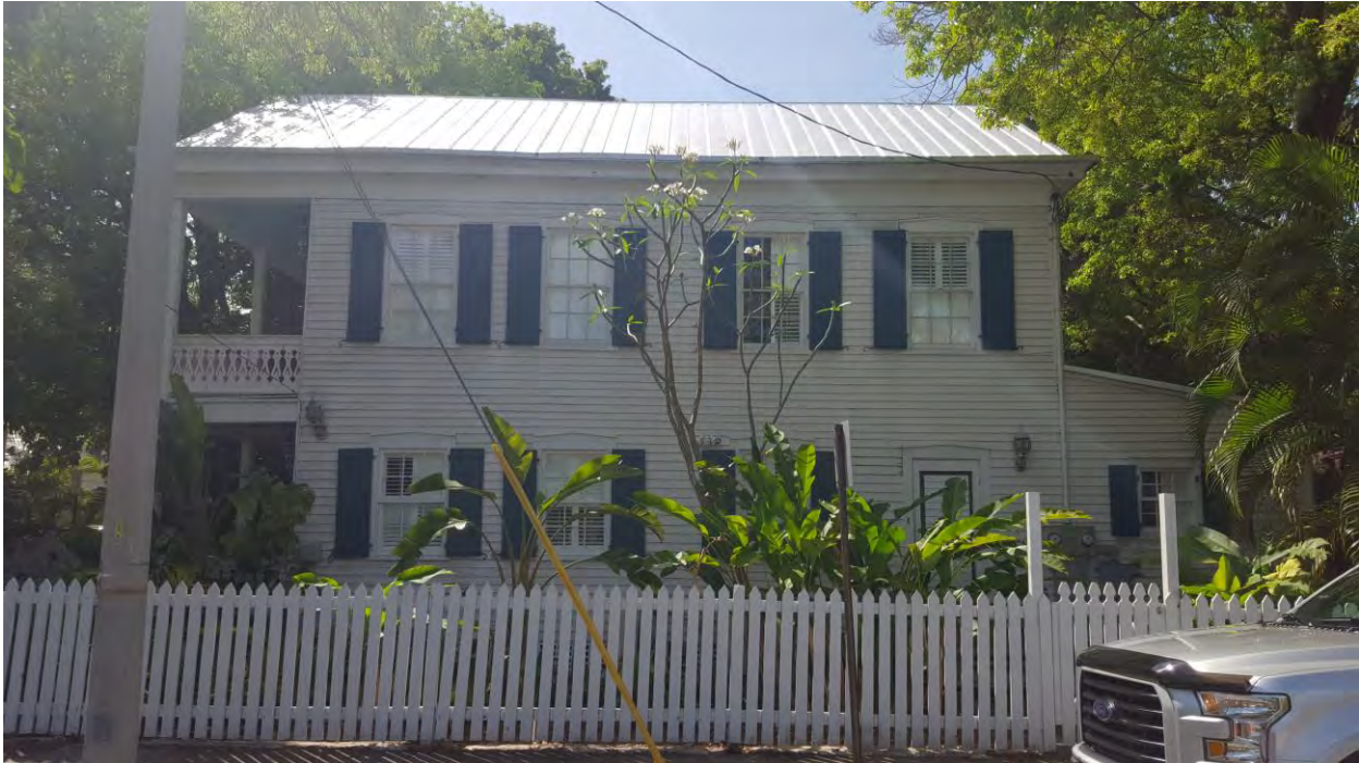
Side of 902 Windsor Lane
