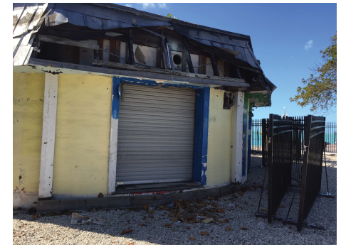
REMOVE ALL EXISTING DOORS AND ROOFING. ALL HISTORIC TIMBERS COLUMNS & BEAMS TO REMAIN AND REPAIRED AS REQUIRED
