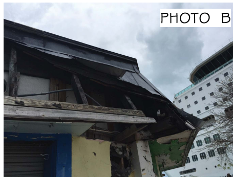
REMOVE EXISTING METAL ROOFING, ROOF FRAMING AND DETERIORATED SOFFIT
