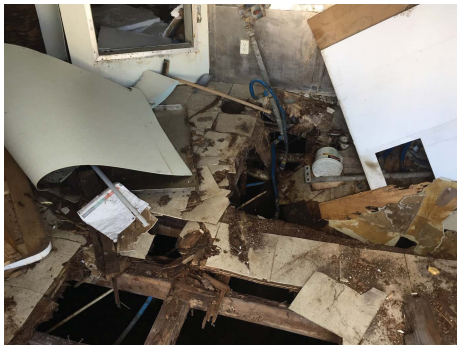
INTERIOR REMOVE DETERIORATED FLOORING AN REPLACE
