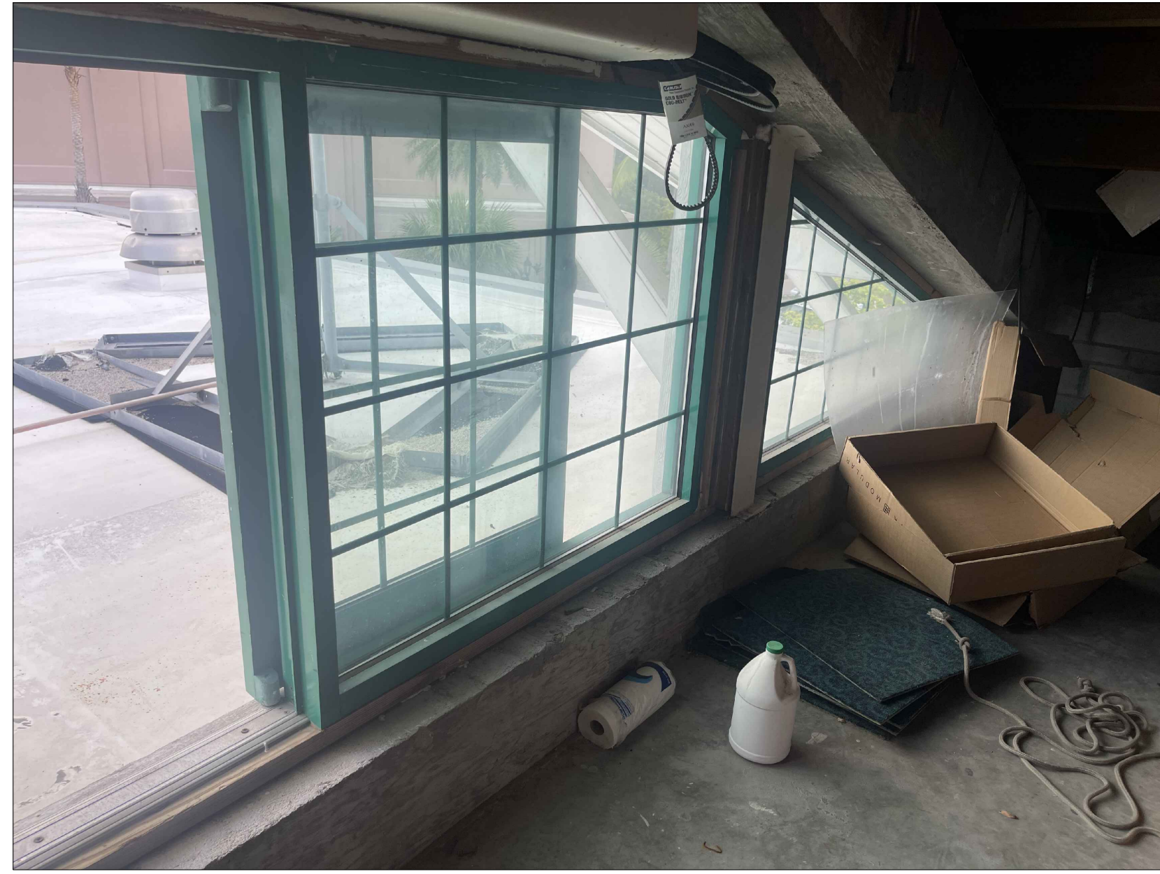
2 ROOF WINDOW PHOTO
