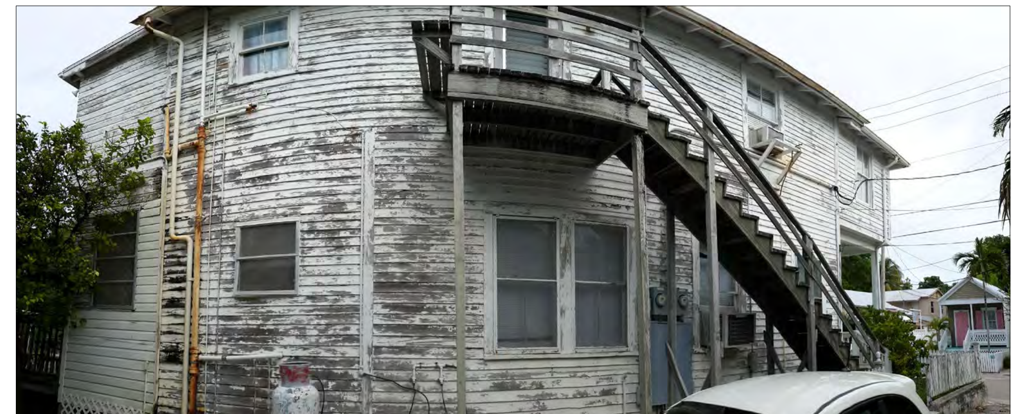
LOOKING NORTHEAST (SIDE)
