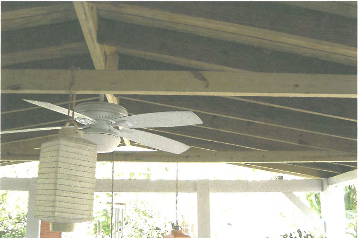
EXISTING FRONT PORCH STRUCTURE LOOKING TOWARD OLIVIA ST.
