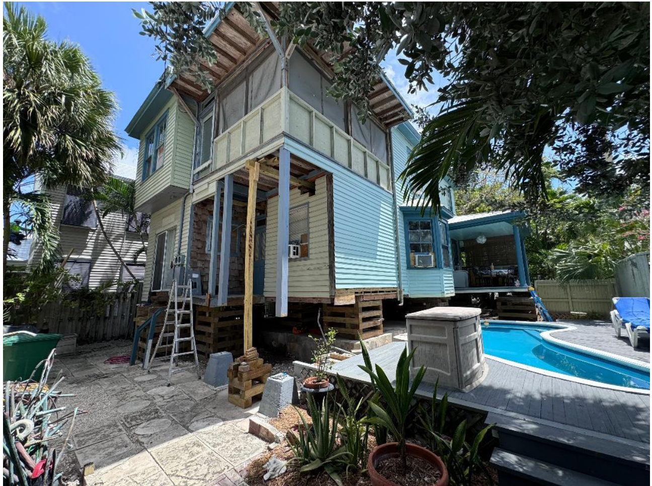
After Lift before North Wall demo
