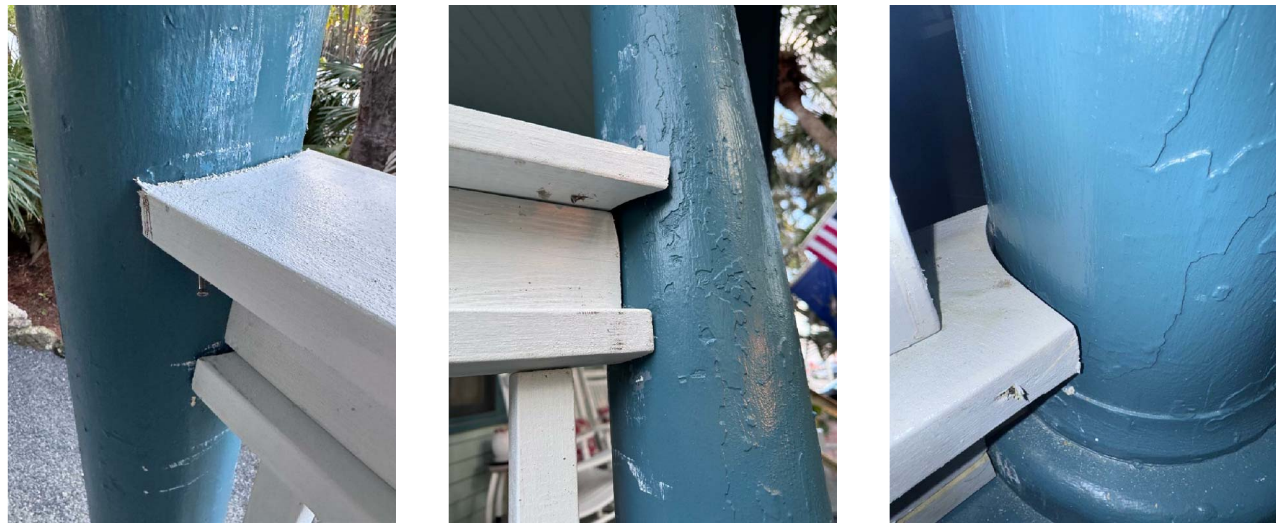
DETAIL - RAILING ATTACHED TO COLUMNS
