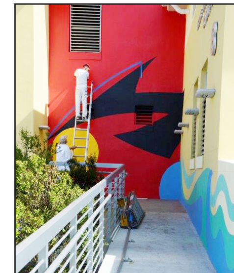
2014 Stock Island Fire Station
