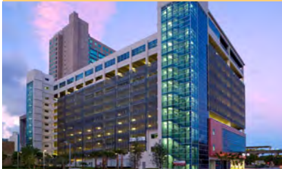
Miami Courthouse Garage, Miami, Florida
