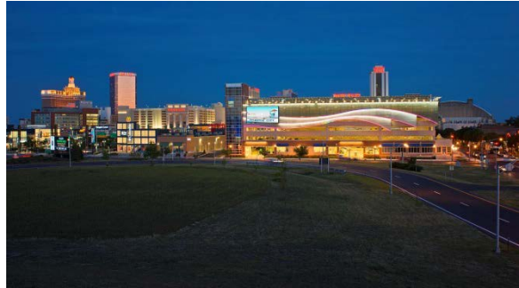
TimHaahs provided prime design services for a new 1180-space mixed-use parking structure in Atlantic City. The garage serves as a "gateway" to the City, and features a number of unique elements including solar panels, metal screens with colored lighting, and LED digital billboard.
