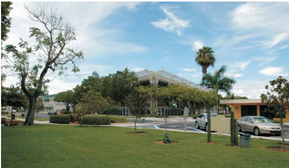
For the City of Naples, TimHaahs provided parking design and structural engineering for a new 328-space public parking facility in downtown Naples.
