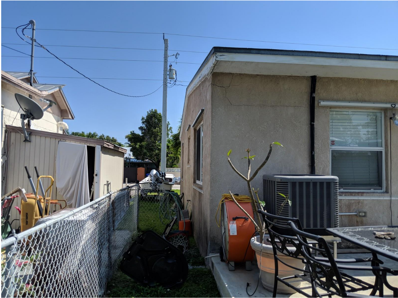
2415 Fogarty Avenue, Key West, Florida 33040 SITE VISIT
