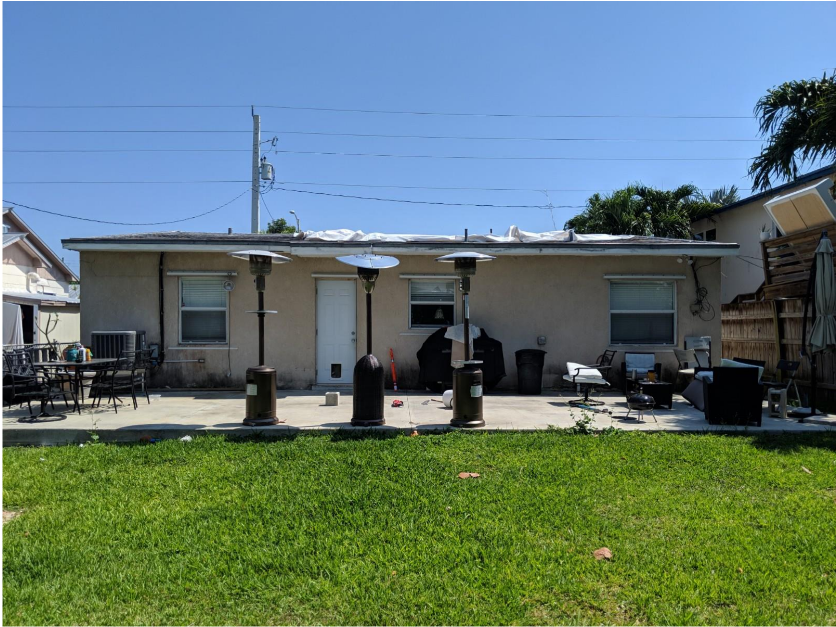
2415 Fogarty Avenue, Key West, Florida 33040 SITE VISIT
