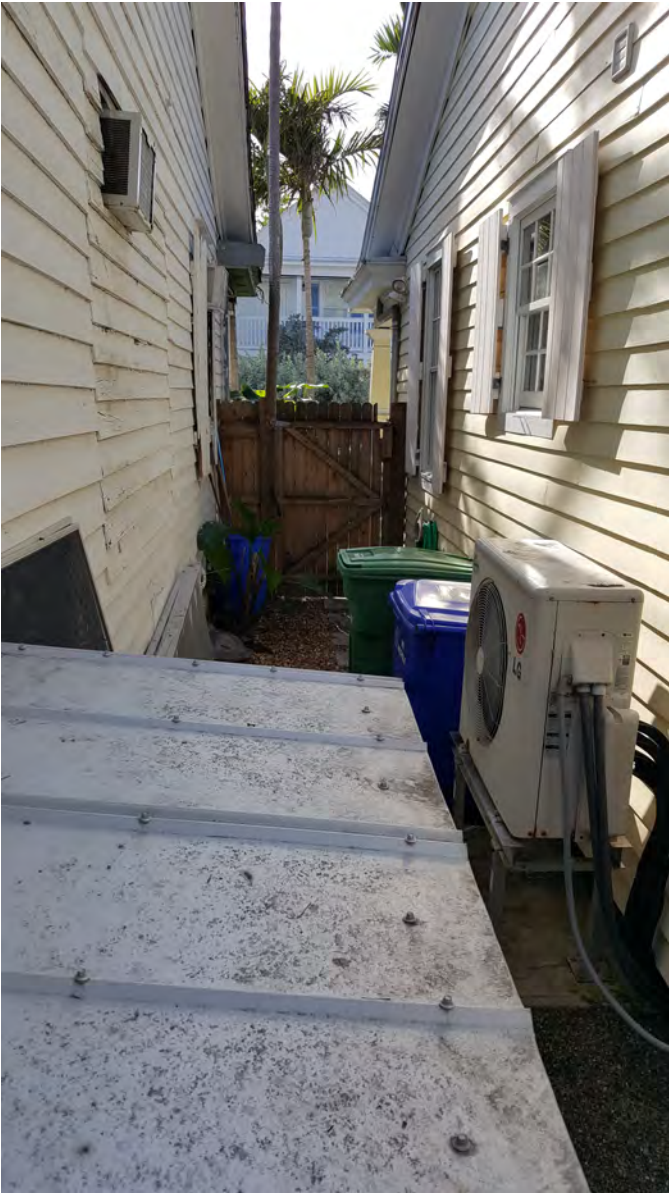
Left-side yard view from rear
