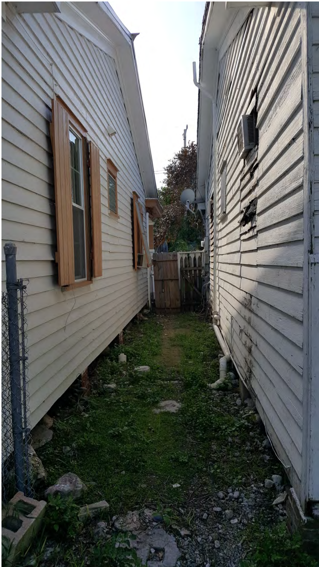
Right-side yard view from rear yard facing towards Whitehead Street
