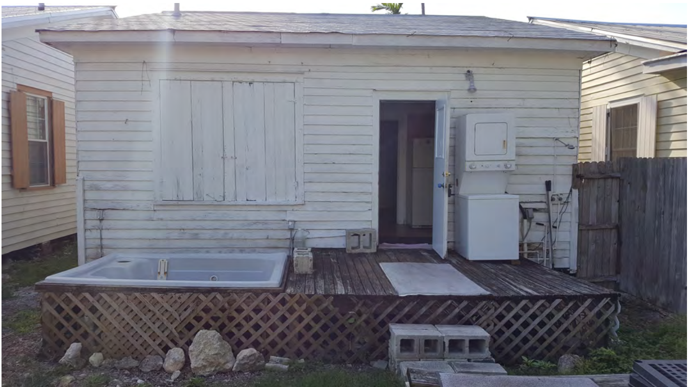
Existing rear wood deck and spa viewed from the rear of the property
