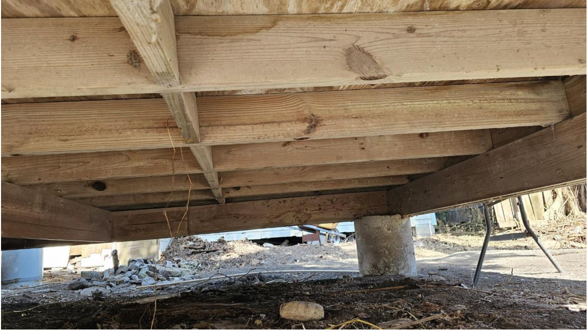
Foundation and underframe of rear addition.
