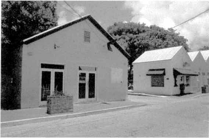
316 Petronia Street (adjacent property)
