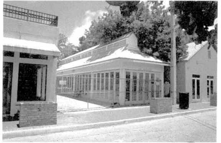
318 Petronia Street (project area)
