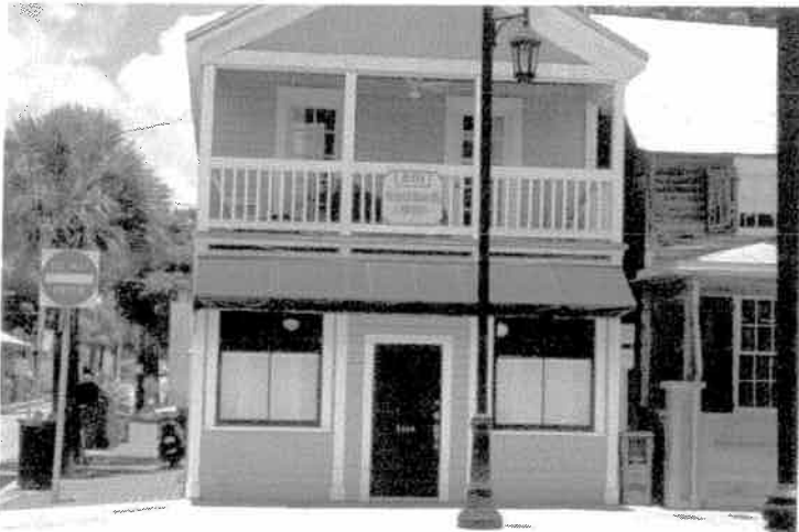
801 Whitehead Street at Petronia Street (neighboring property)
