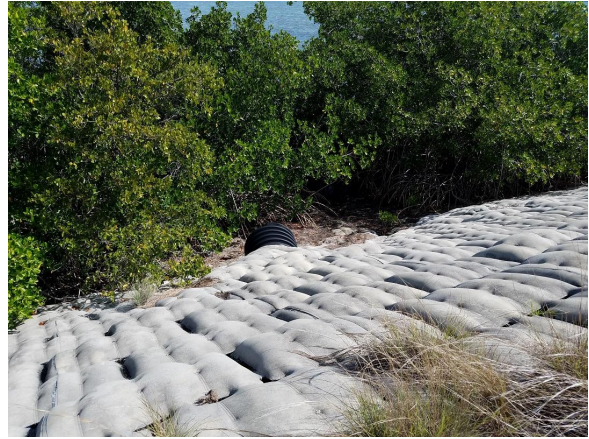
Stormwater outfall
