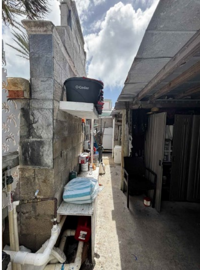
Existing Accessory Structure (East Elevation)
