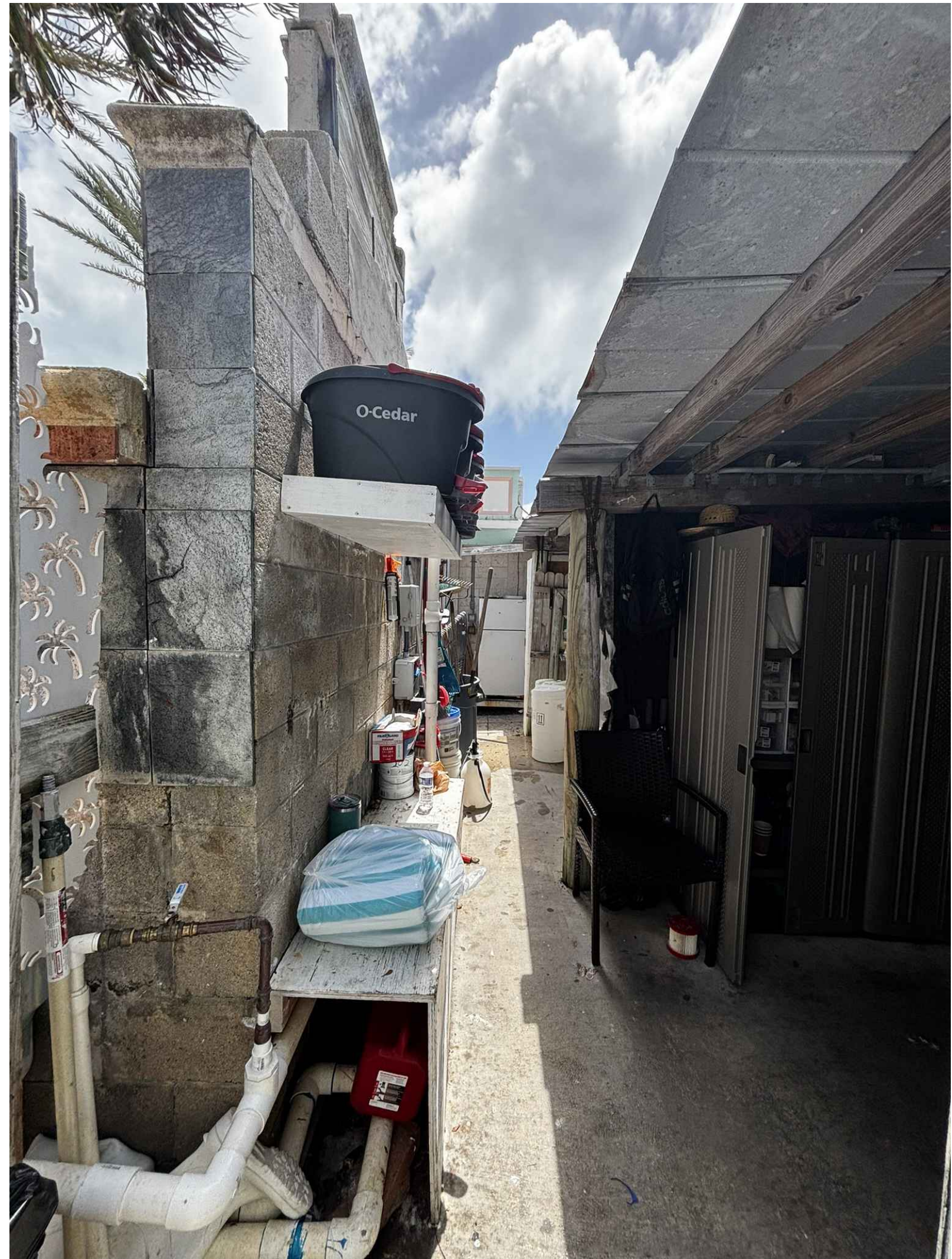
3 PHOTOGRAPH OF EXISTING STRUCTURE (EAST VIEW) A4 SCALE: N.T.S.
