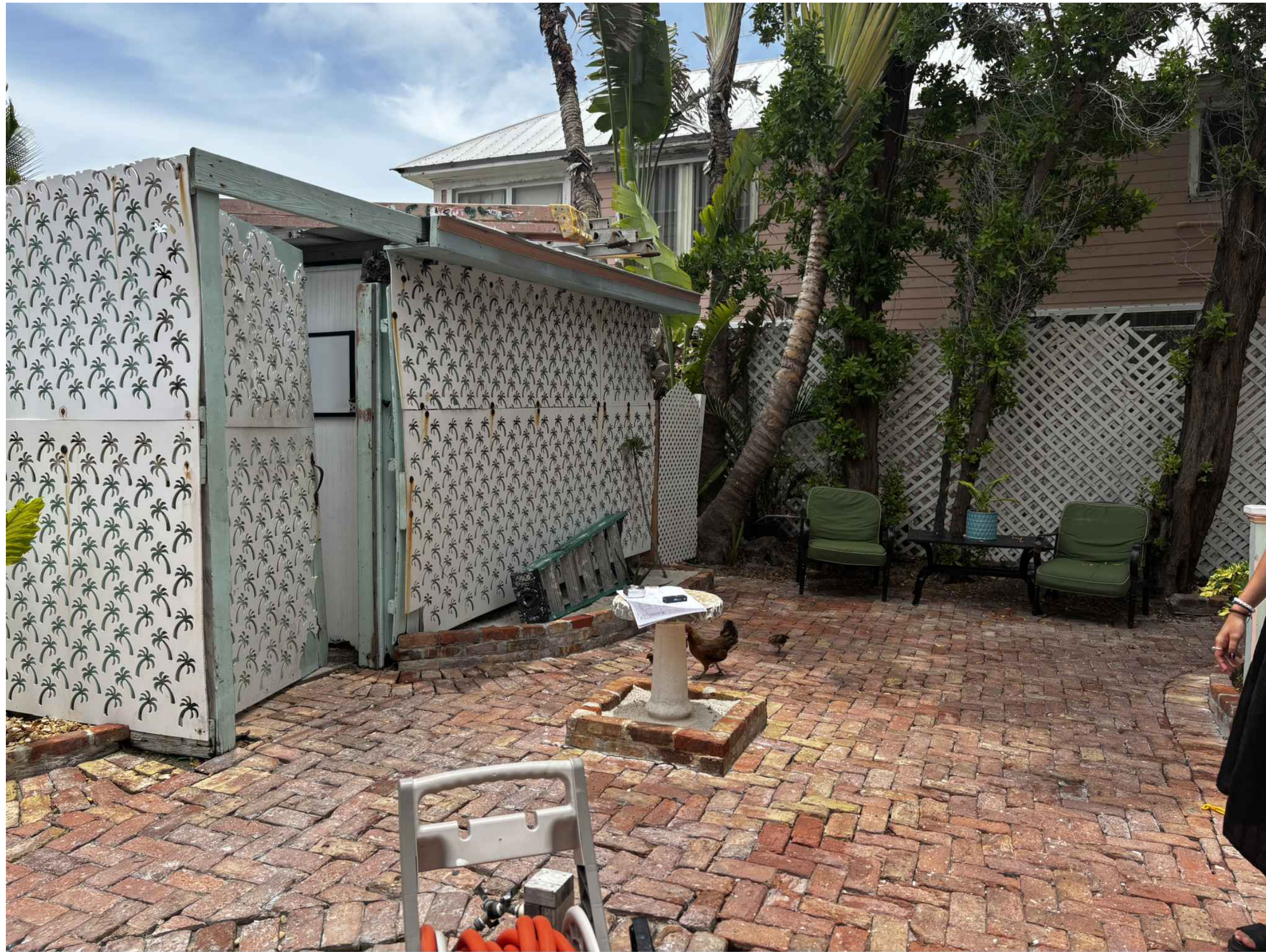
4 A4 PHOTOGRAPH OF EXISTING STRUCTURE (NORTH VIEW) SCALE: N.T.S.
