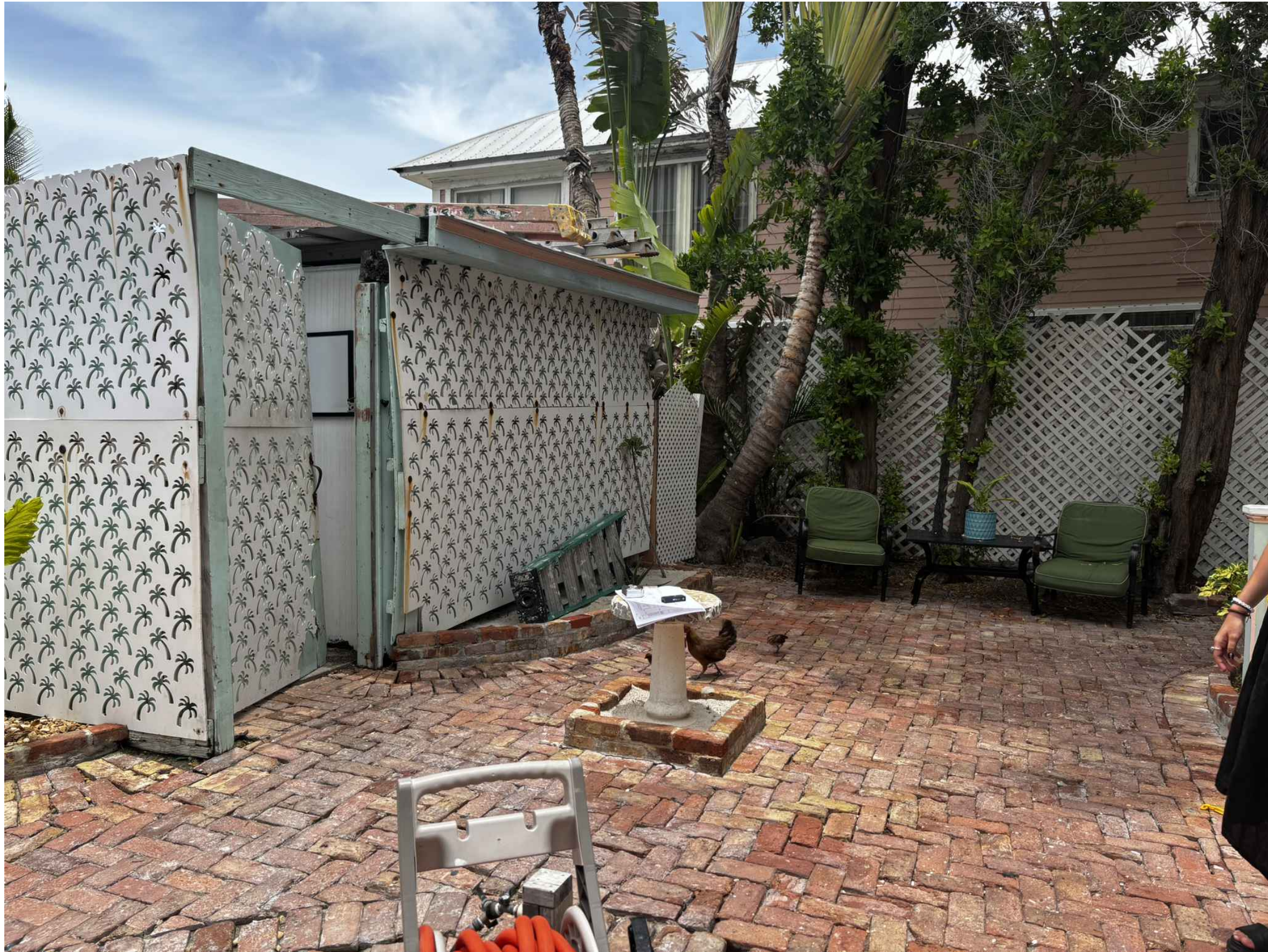
4 PHOTOGRAPH OF EXISTING STRUCTURE (NORTH VIEW) A4 SCALE: N.T.S.
