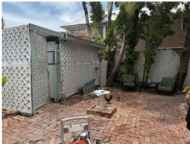
Photo of Existing Structure (North Elevation).
