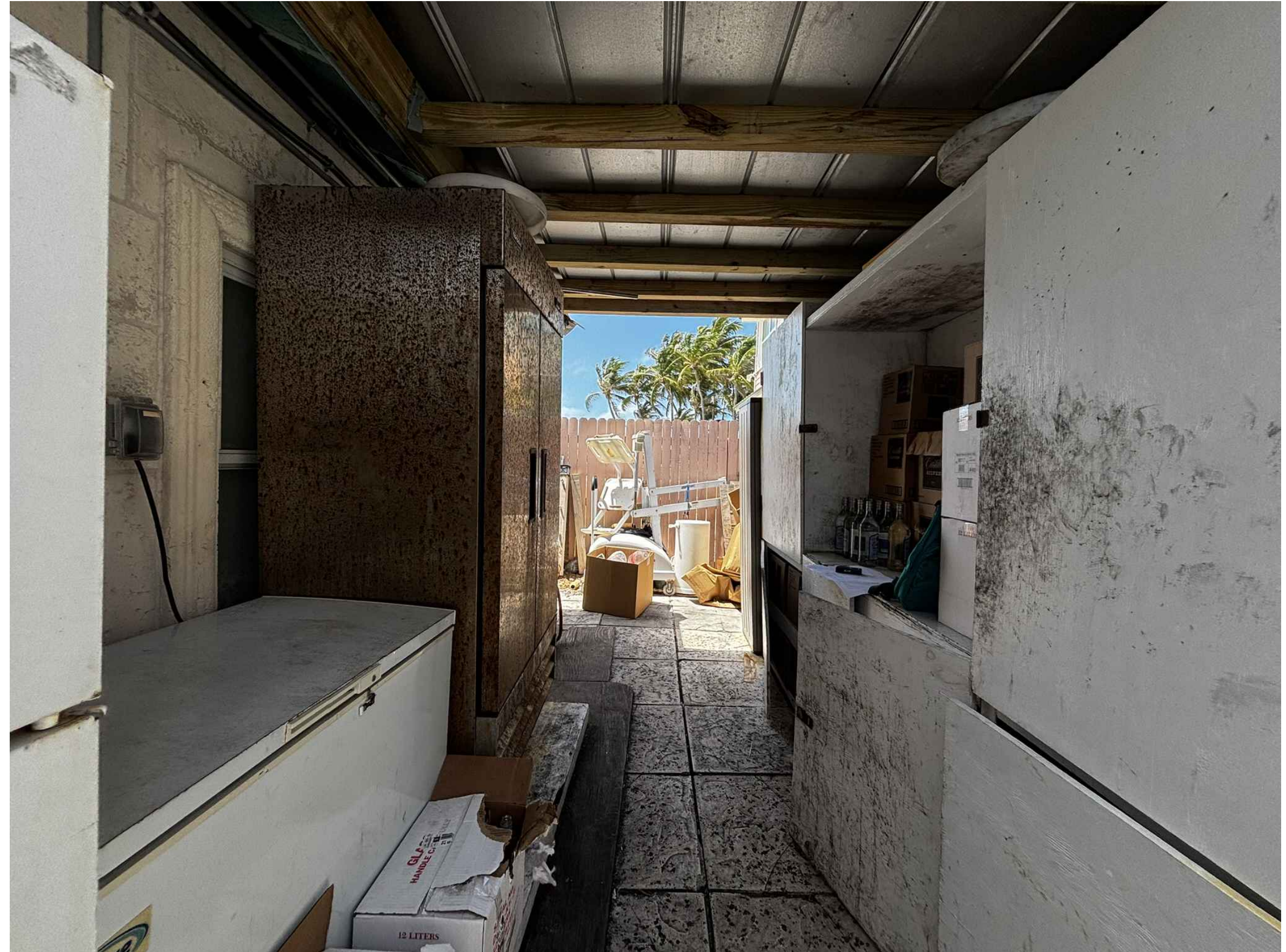
1 PHOTOGRAPH OF EXISTING STRUCTURE (SOUTH VIEW) A4 SCALE: N.T.S.
