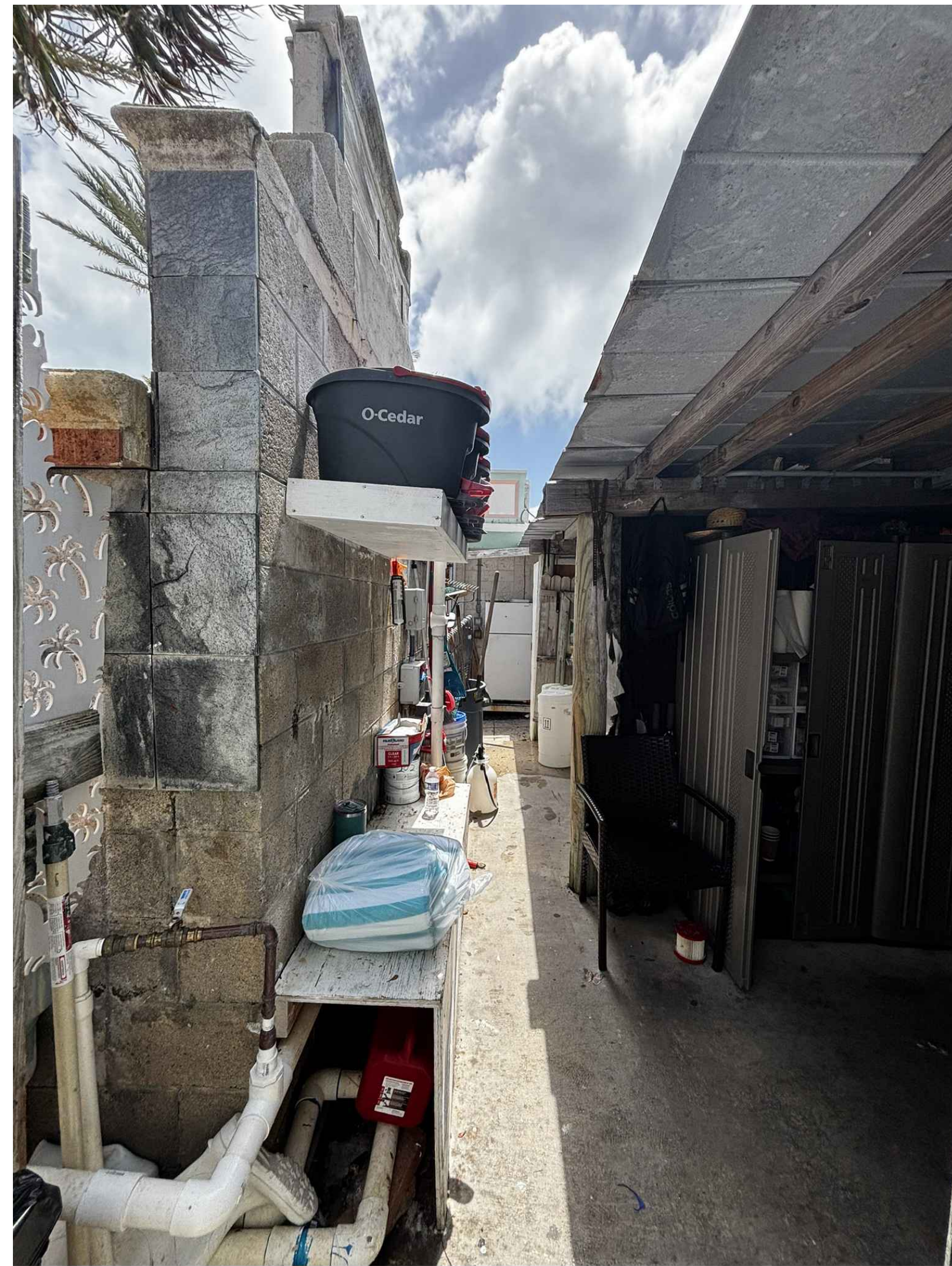
3 A4 PHOTOGRAPH OF EXISTING STRUCTURE (EAST VIEW) SCALE: N.T.S.
